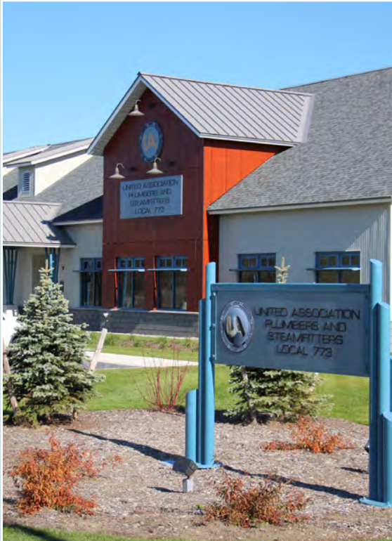
Plumbers and Steamfitters Local 773 in Glens Falls.
