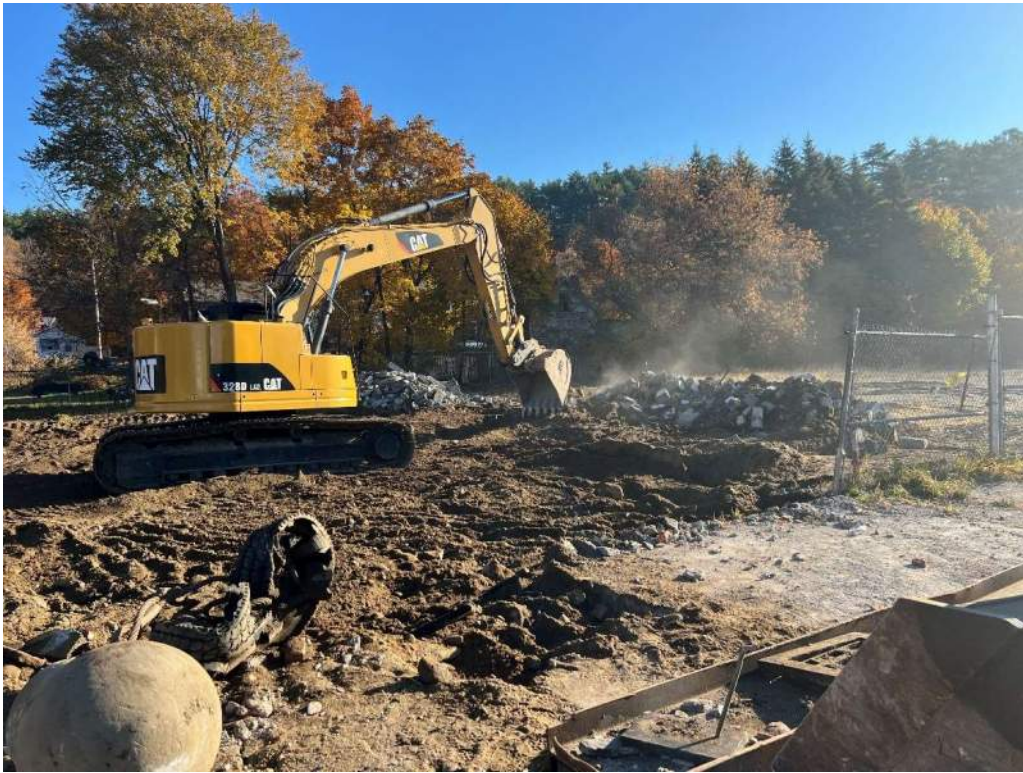
Tank A Area
