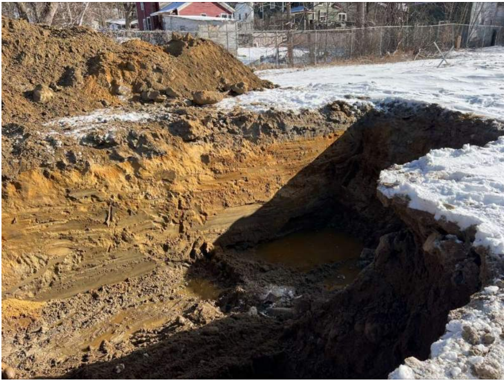
Tank B Soil Excavation 1.28.2025
