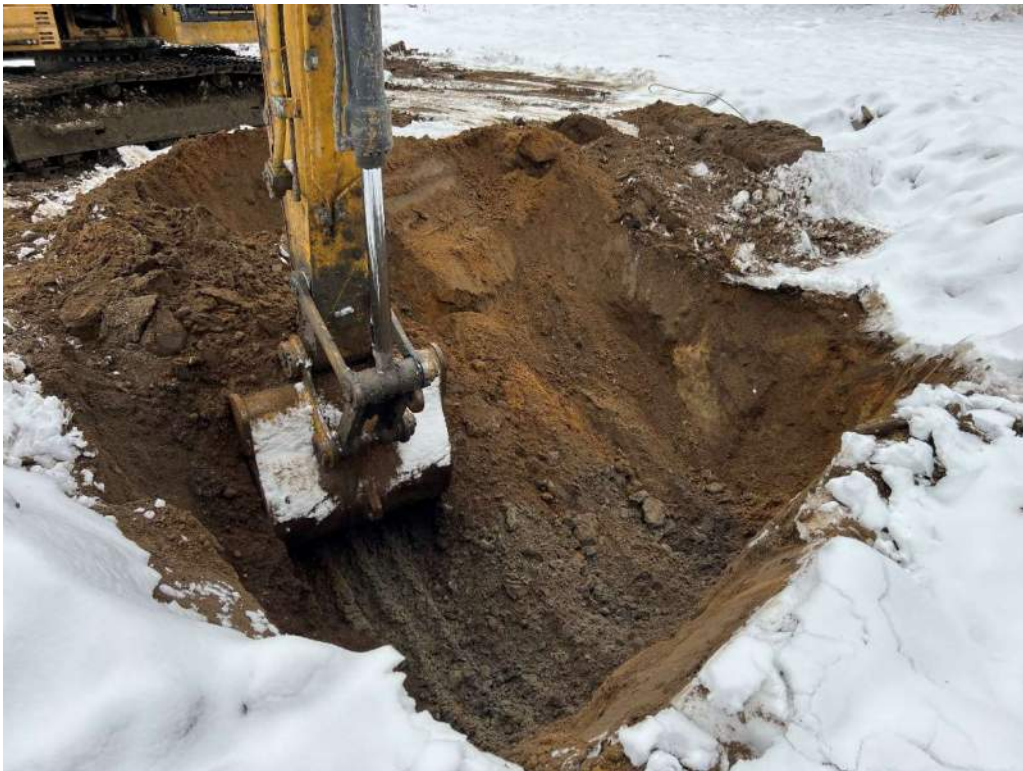
Tank B Soil Excavation 12.10.2024
