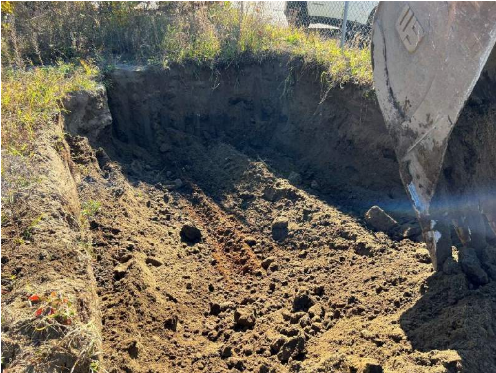
GPR Anomaly - Pipe & Tile Fragments
