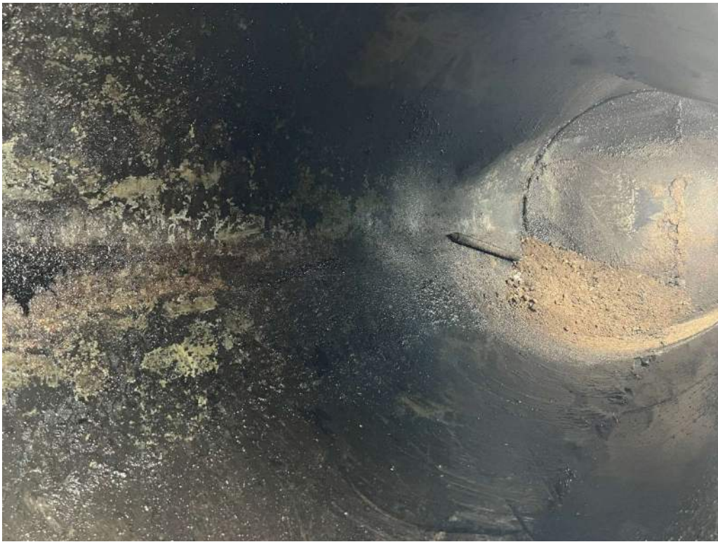
Tank B Interior
