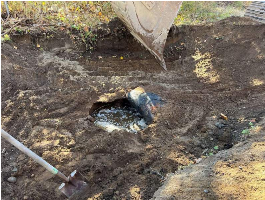
GPR Anomaly - Septic Tank
