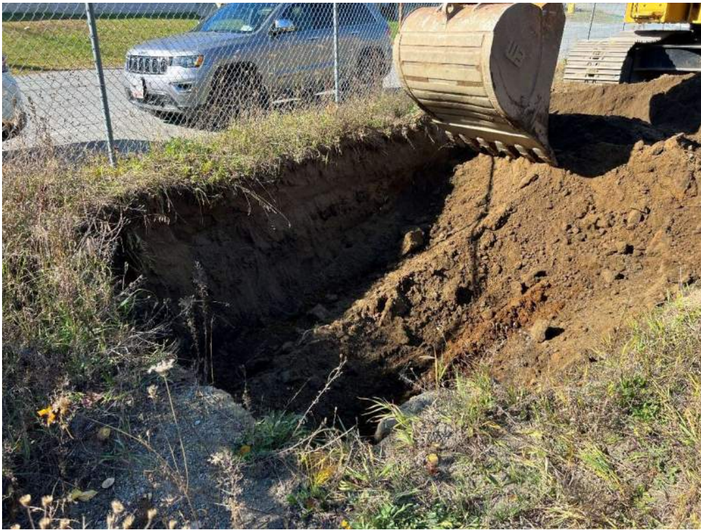
GPR Anomaly - Pipe & Tile Fragments
