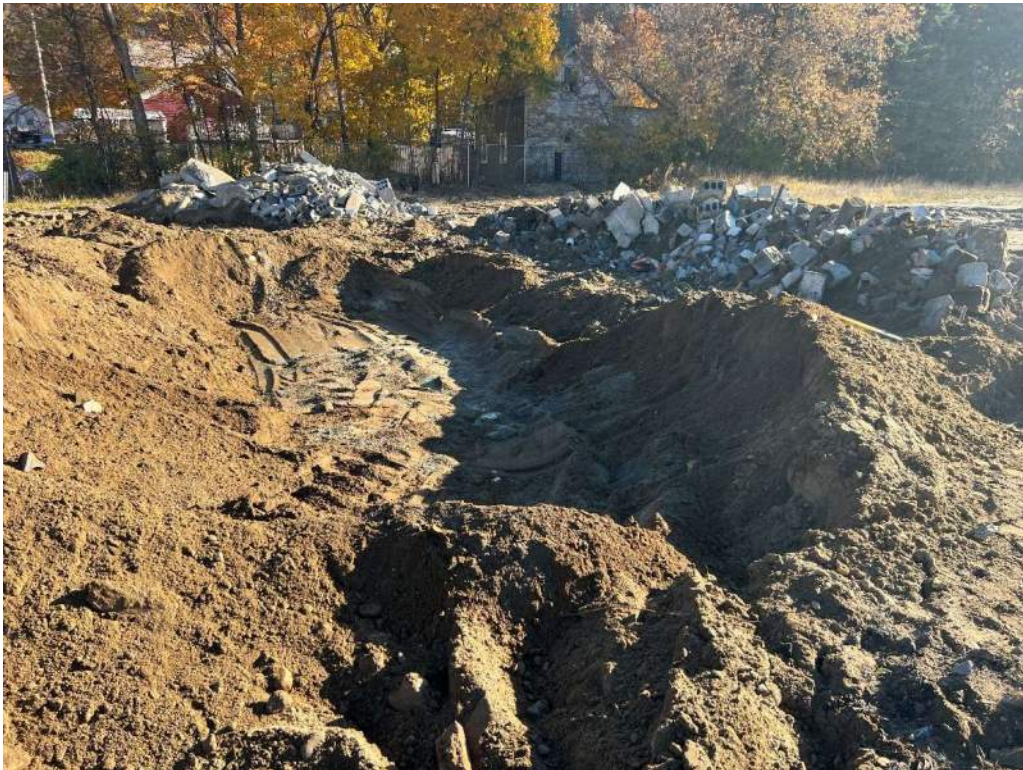
Tank A Area
