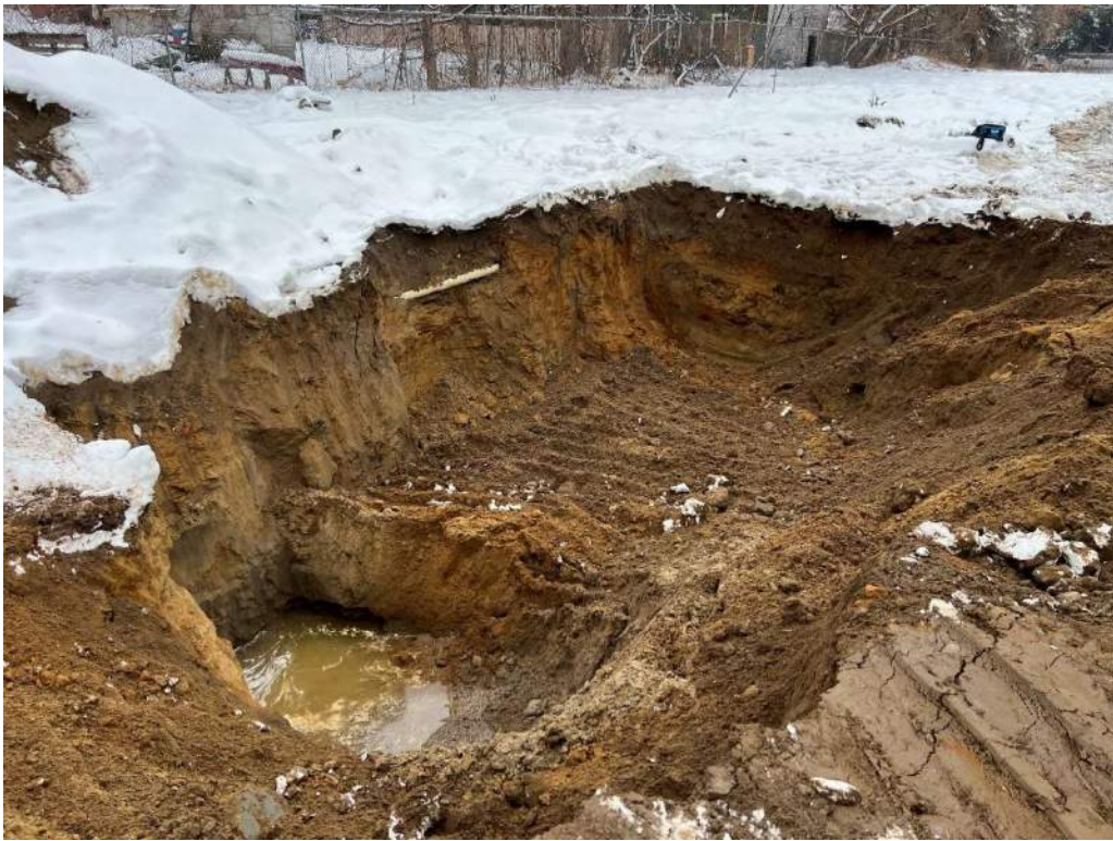
Tank B Soil Excavation 12.10.2024
