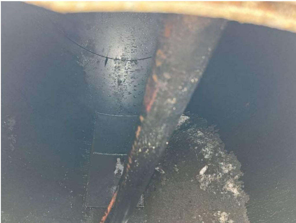
Tank A Interior
