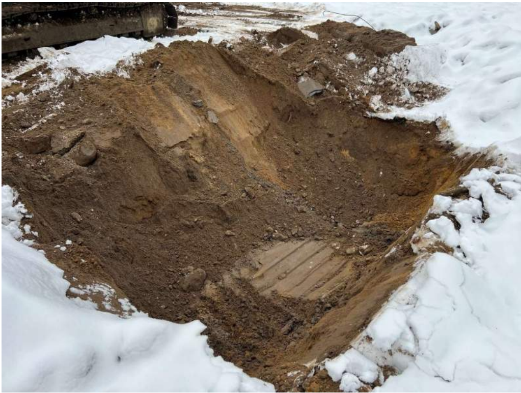
Tank B Soil Excavation 12.10.2024
