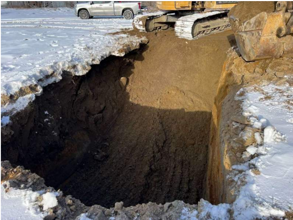
Tank B Soil Excavation 1.28.2025
