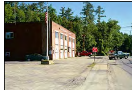
Building Facade Detracts From Gateway Image
