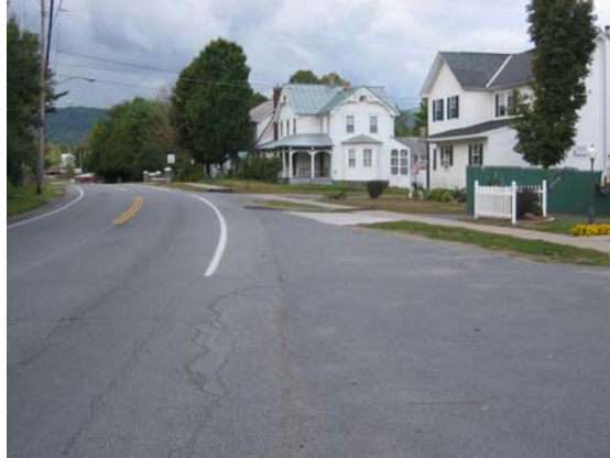
Image 9: The view of Rockwell Street approaching Hadley from Fowler Park shows the current condition with excessive paving, deteriorating curbs, and overhead wires (Appendix C, Hadley Center & Rockwell St. Improvement Plan).
