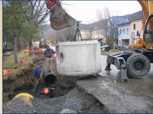
Stormwater collection equipment being installed along West Brook Road
