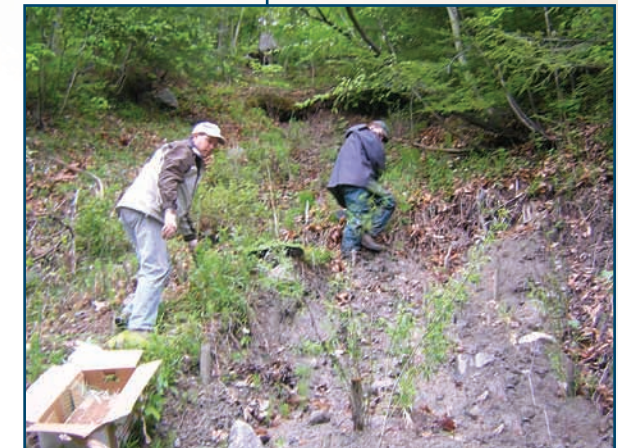
Installation of sedimentation vegetation by WCSWCD along Hague Brook
