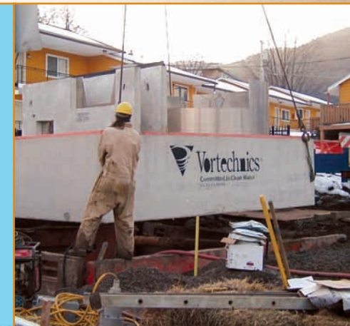
Vortechics unit being installed
