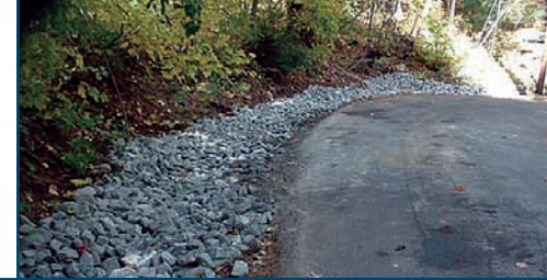
Stormwater improvements installed along roadway at Pioneer Village-Bolton
