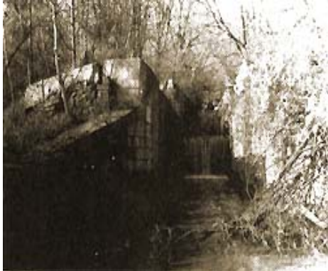
Combination locks on the Feeder Canal
