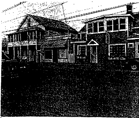
Figure 21. Historic facades on Main Street North Creek, circa 1992.
