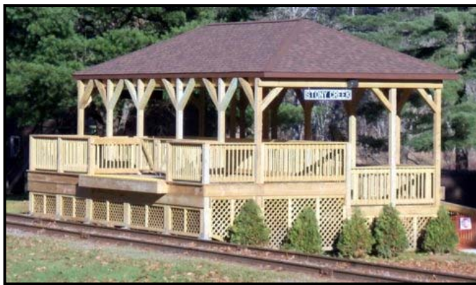
Figure 16: Town of Stony Creek platform rail station at 1000 Acres. Courtesy of P. Morin
