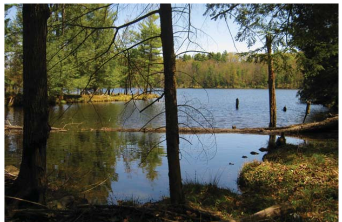
All Photos are Edgecomb Pond, Photo credit: C.T. Male (dam)
