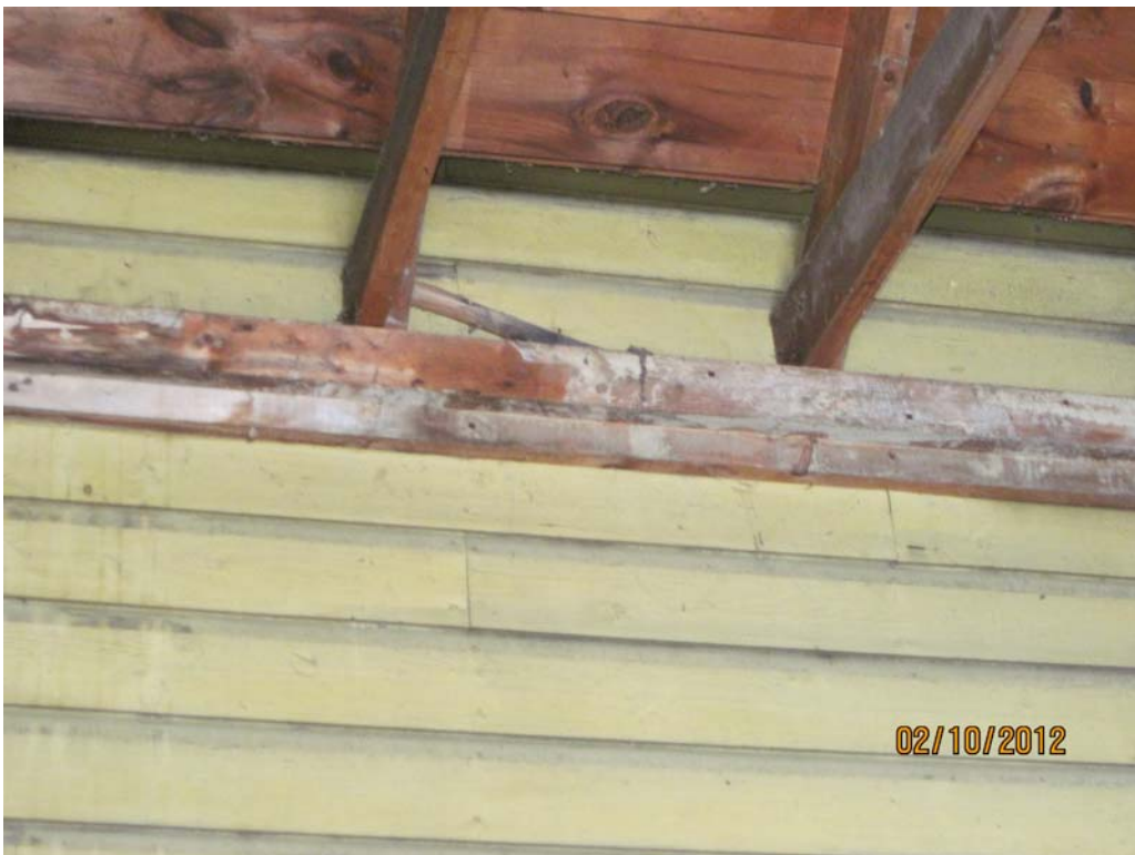
Photograph 33 – “T” Building – Connection of Addition Roof Framing to Main Building
