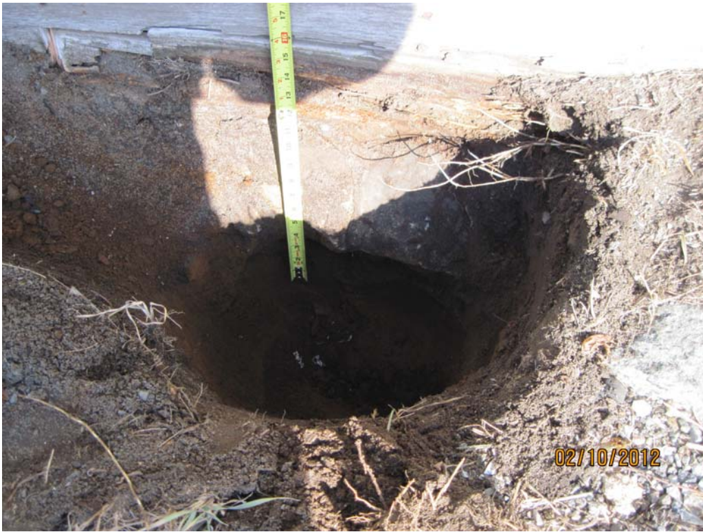
Photograph 7 – Stables Stone Foundation
