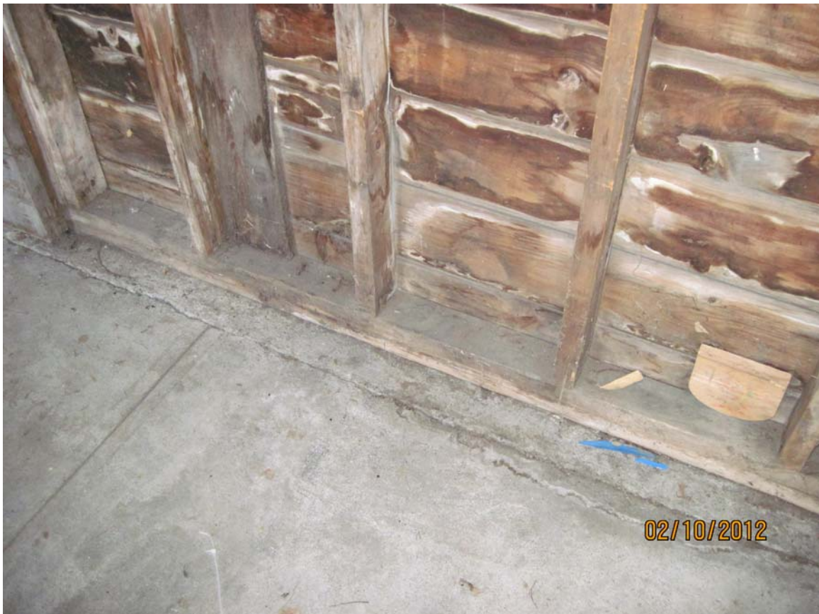
Photograph 31 – “T” Building – Bottom of Floor Framing in Addition
