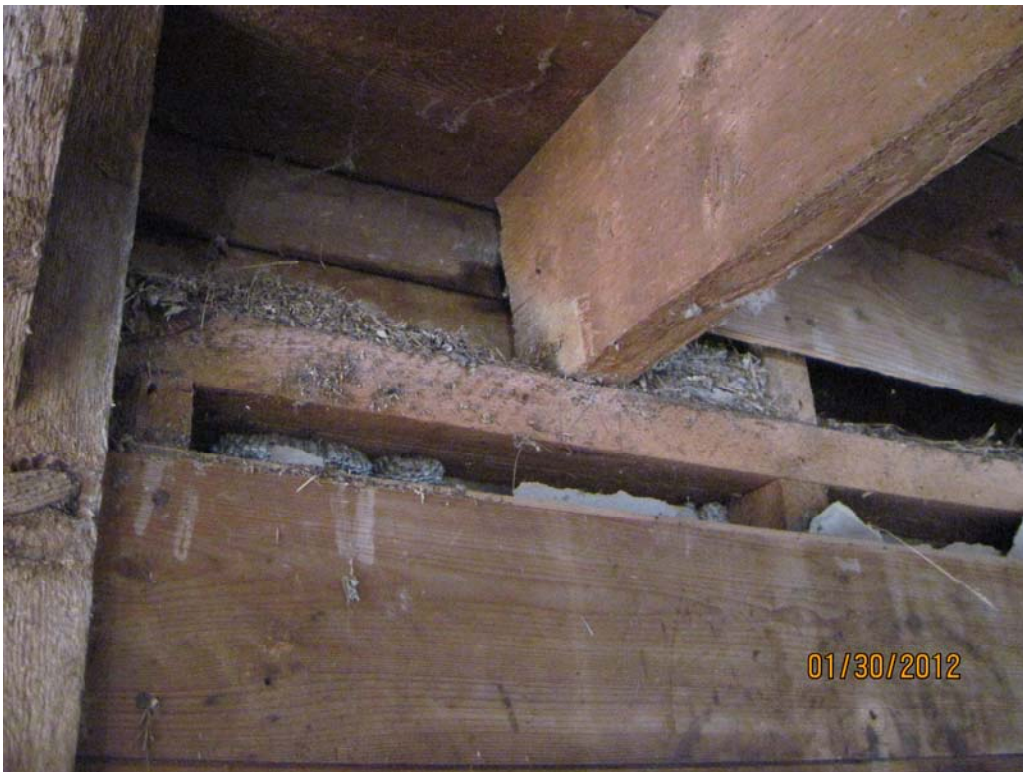
Photograph 6 – Stables Bearing of Loft Floor Joist on Wall Plate
