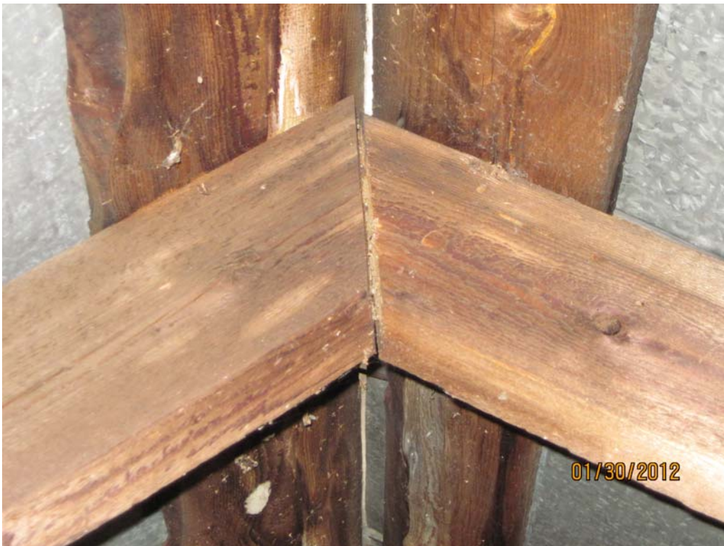
Photograph 2 – Stables Typ. Rafter at Ridge
