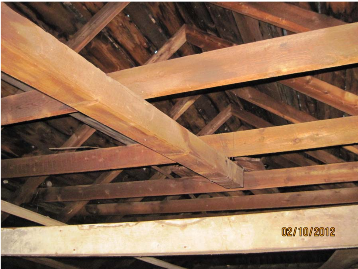
Photograph 14 – Scales Building Rafters with Hoist Beam Tied to Collar Tie
