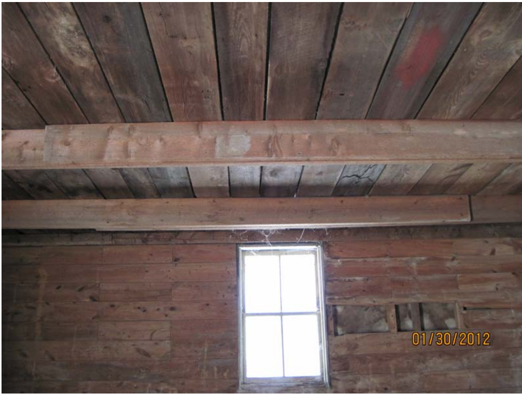
Photograph 5 – Stables Loft Floor Joist Construction
