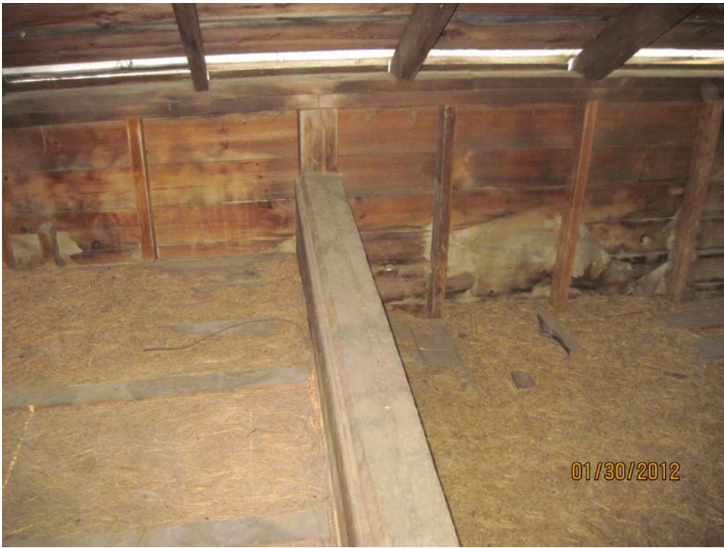
Photograph 3 – Stables Typ. Tie Beam and Upper Wall Construction
