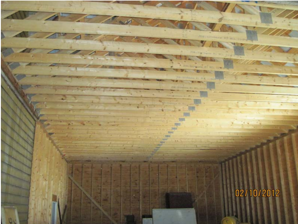
Photograph 32 – “T” Building – New Truss Framing in Addition
