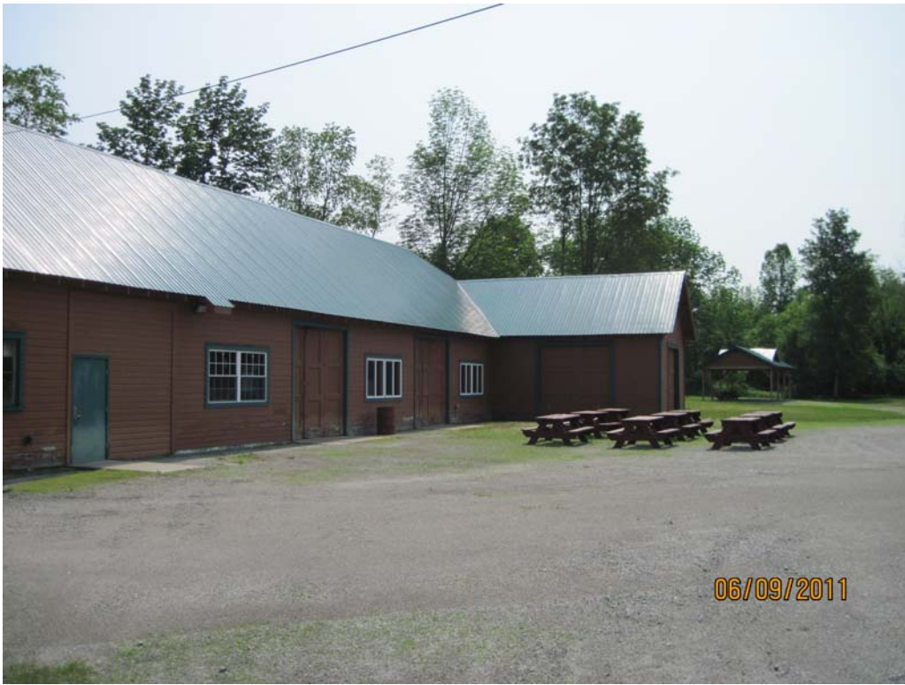
Photograph 26 – “T” Building – West Elevation, Note Height of Outside Grade Elevation
