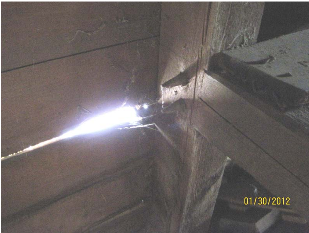
Photograph 4 – Stables Mortise and Tenon Joint at Tie Beam
