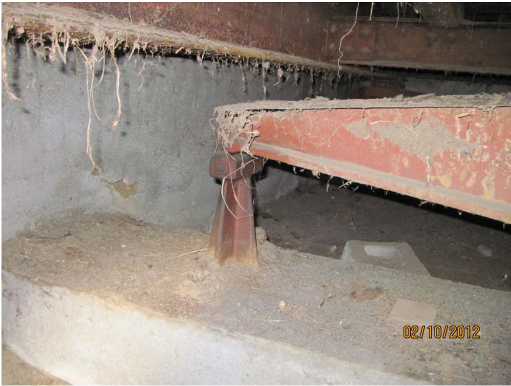
Photograph 21 – Scales Bldg. – Scale Pit Mechanism Bearing on Concrete Pier
