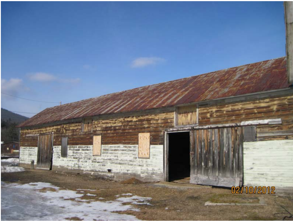
Photograph 1 – South Elevation of Stables Building
