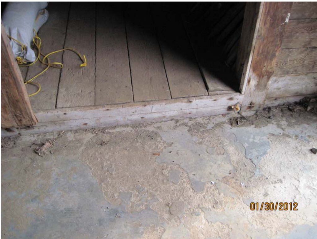
Photograph 8 – Stables Transition of Wood Floor to Concrete Slab
