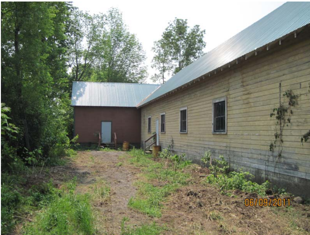
Photograph 27 – “T” Building – East Elevation with Addition in Background
