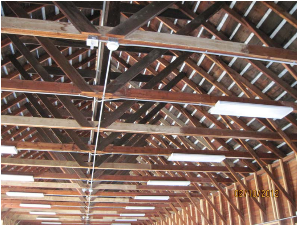
Photograph 28 – “T” Building – Main Building Rafter and Truss Framing
