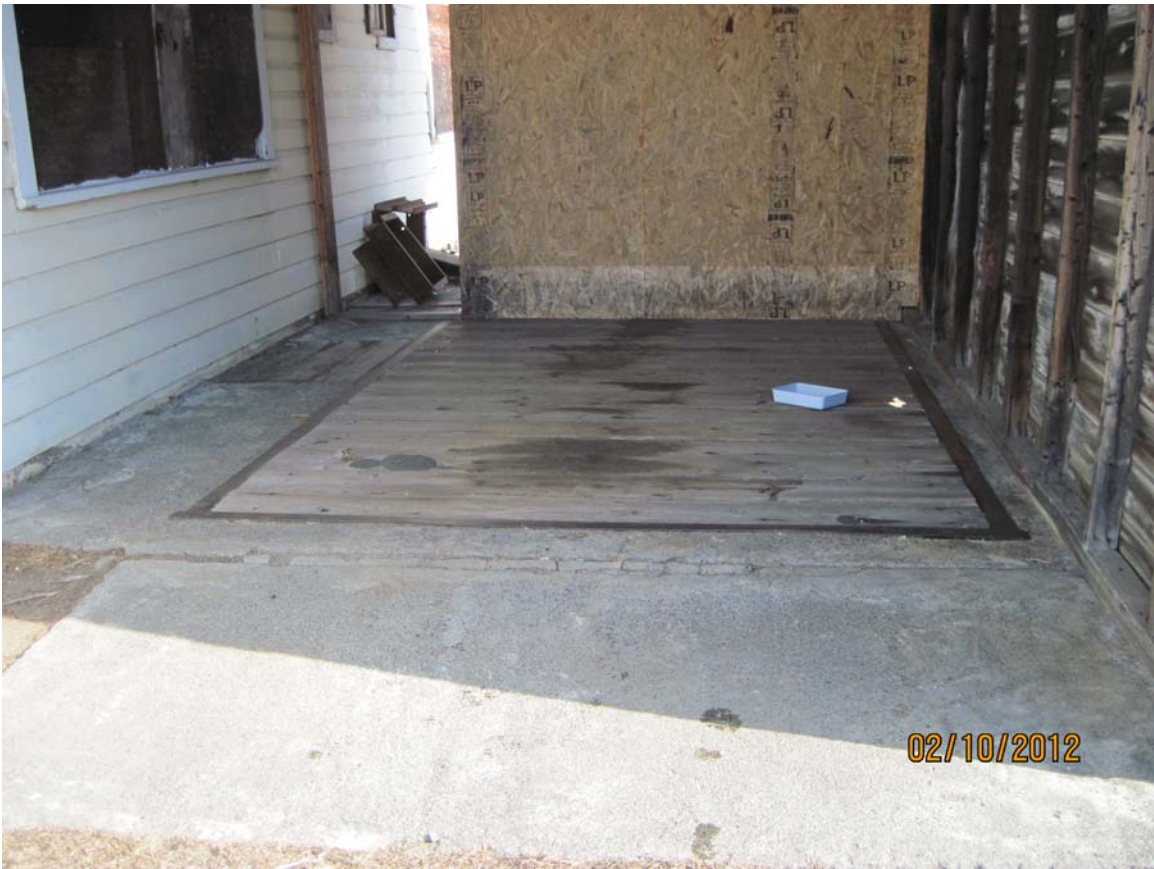
Photograph 23 – Scales Bldg. – Scale Pit Flooring w/ Enclosure Support Wall on Right
