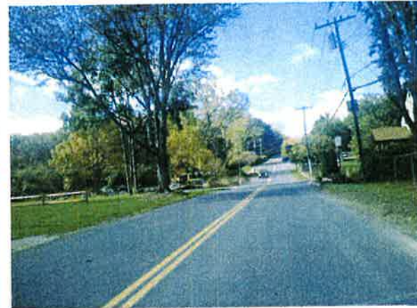
Murray St. – lack of designated shoulders (Looking west towards Murray St. Park)
