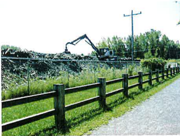
Light industrial uses along Feeder Canal Trail
