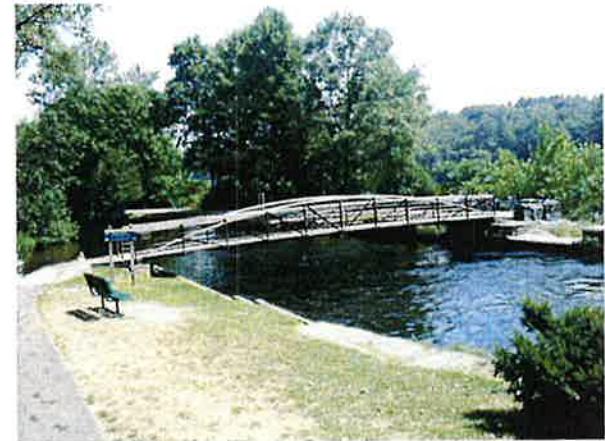
Dual use Bridge at Feeder Canal Park, Queensbury
