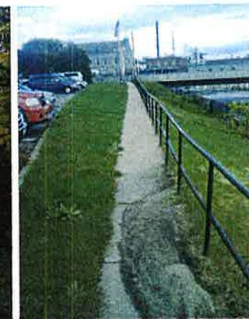
Narrow sidewalk at Glen St. trailhead
