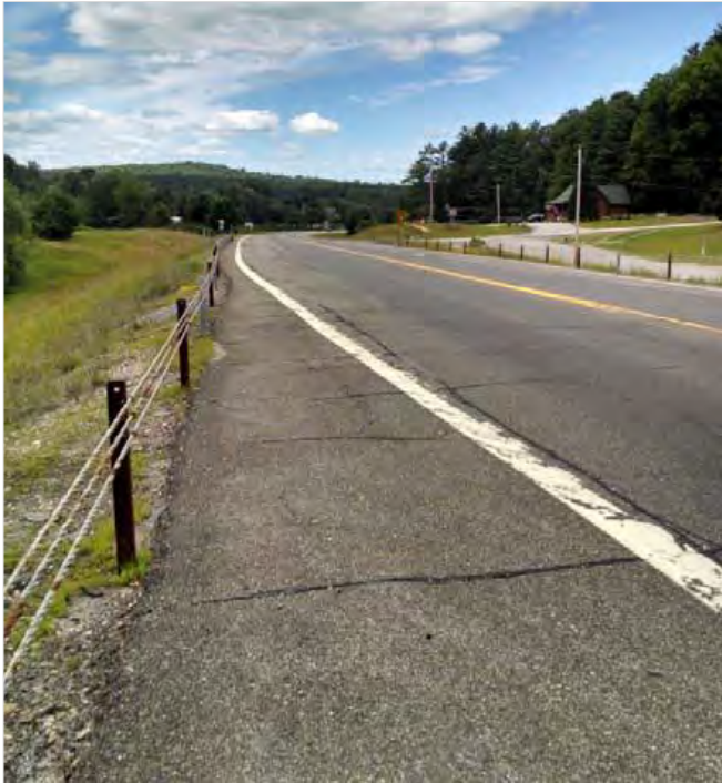
Route 8 Shoulder near Dynamite Hill Recreation Area
