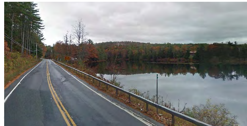
Western portions of the River Street corridor is predominantly defined by a more rural characteristic (courtesy Google Street View)
