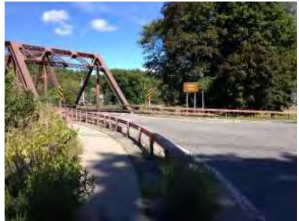
Bridge at Richards Ave. View northeast
