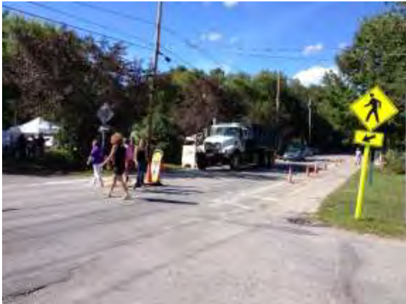
Intersection of River St. and Commercial Ave. View north
