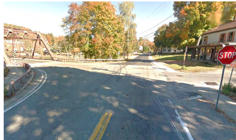
Poor striping, no stop lines, lack of crosswalks, wide turning radii, and an awkward stopping configuration make for seemingly unsafe intersection (courtesy of Google Street View)
