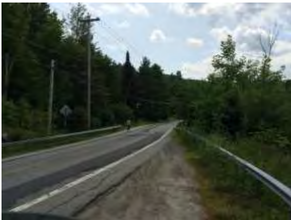
At pull off near substation View west
