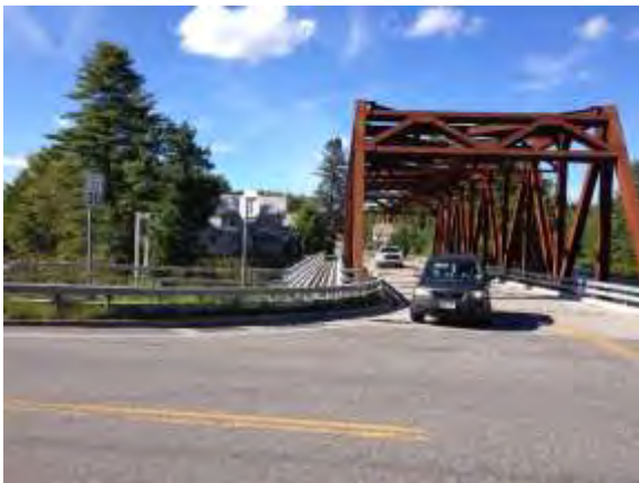
Bridge at Milton St. View north
