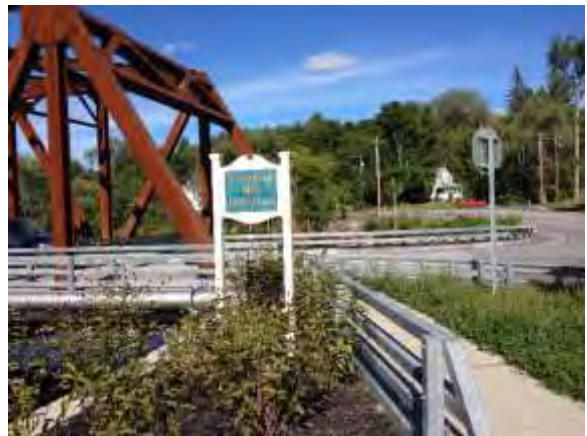
Bridge at Milton St. View east
