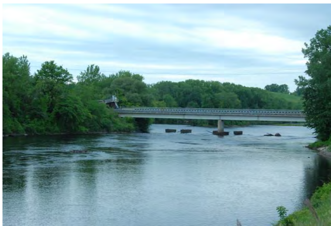
View of Hudson River from Ciba-Geigy Site (looking west)
