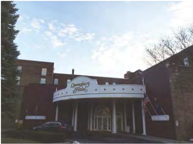
Queensbury Hotel Entry
