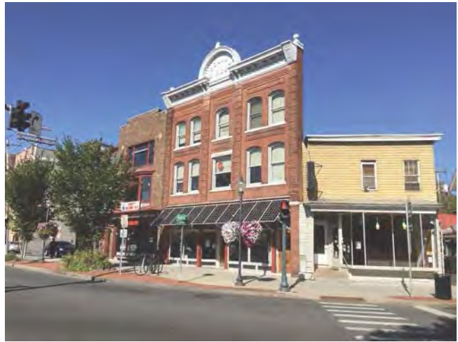
Buildings on South Street and Broad Street
