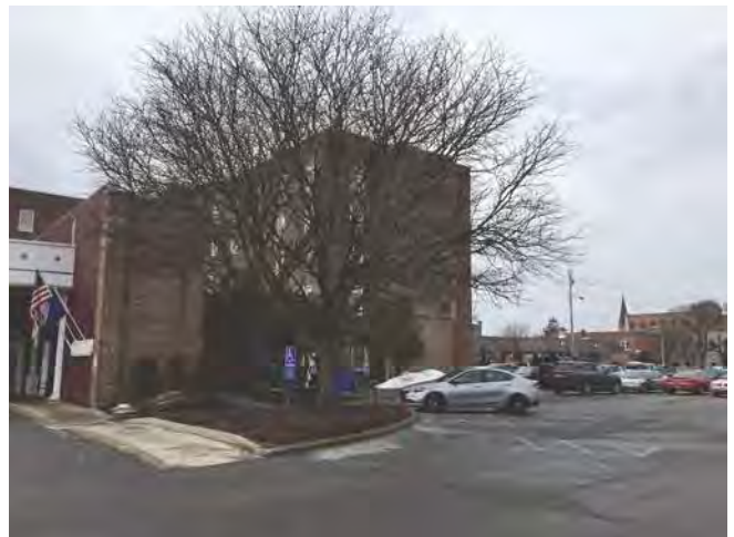
Site of Adirondack Room Expansion
