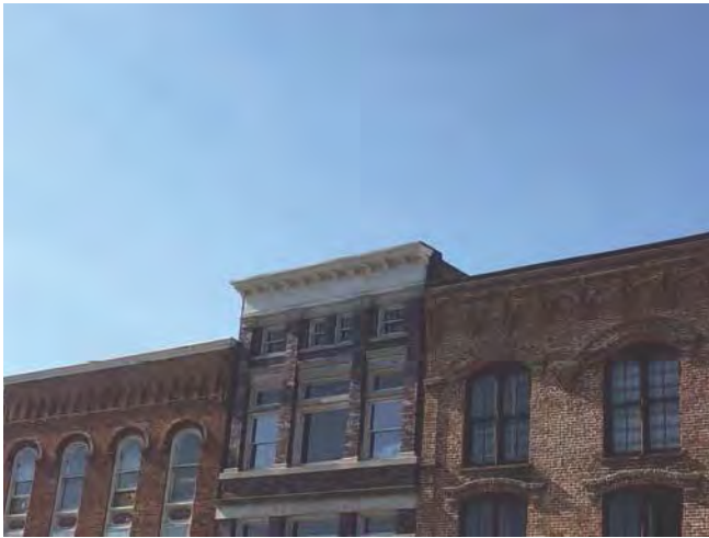
Cornice on Glen Street
