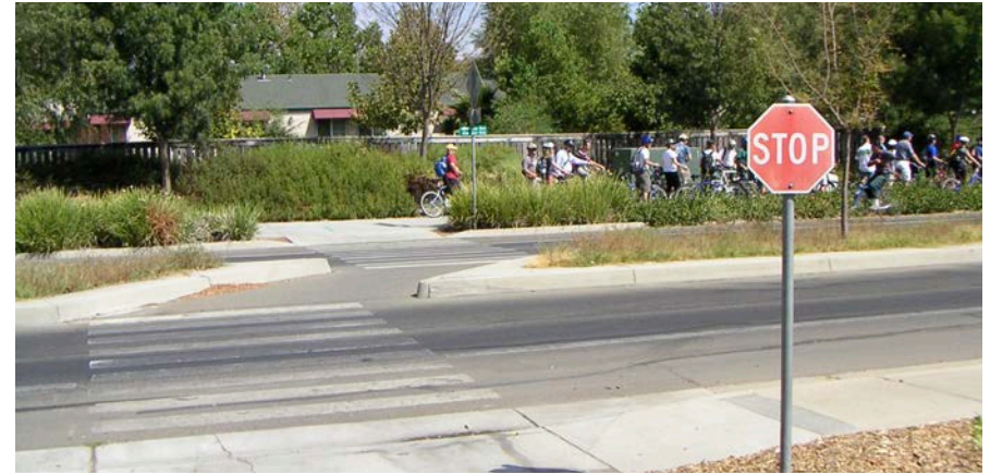
Median refuge islands can have angled passages to orient path users to face oncoming traffic.
