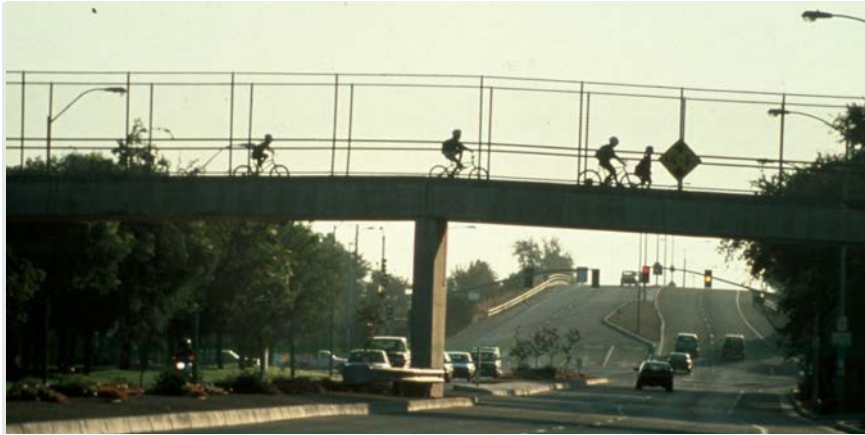
This overpass helps children cross a busy street at a midblock location.
