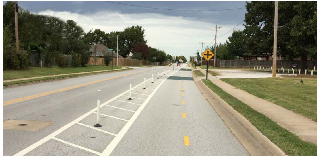
Some segments of the Razorback Greenway Trail operate in the roadway, with minor physical separation between the roadway and the trail.
