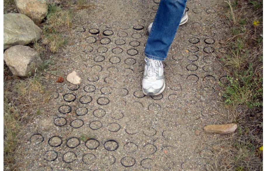
Trail surface material can be further stabilized with a variety of products (Source: National Trails Training Partnership)
