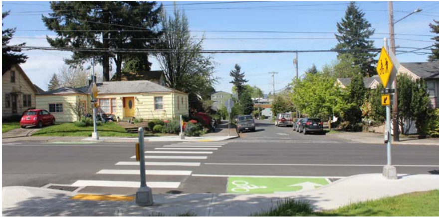
RRFB bikeway crossing with separate push buttons for pedestrians and bicyclists.
