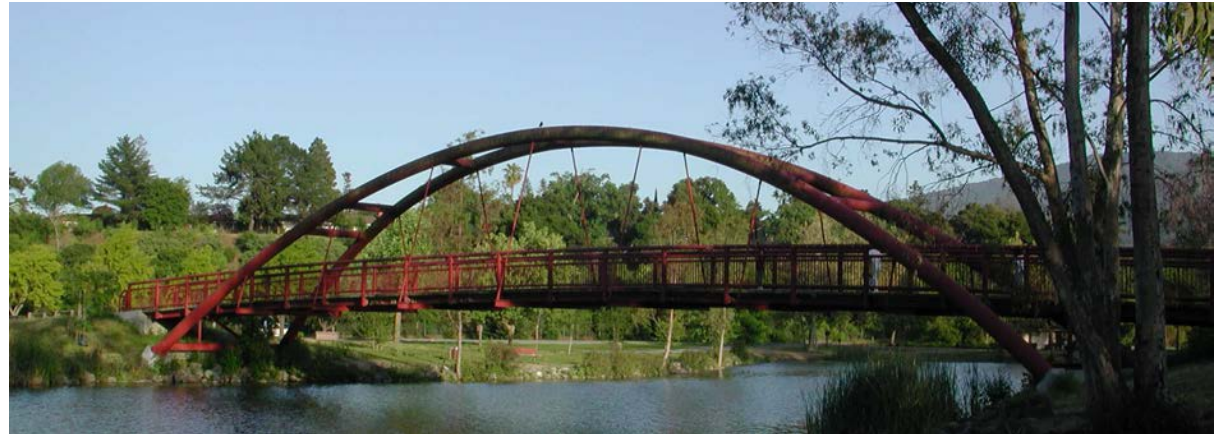
Vasona Lake County Park Bridge, Los Gatos, CA
