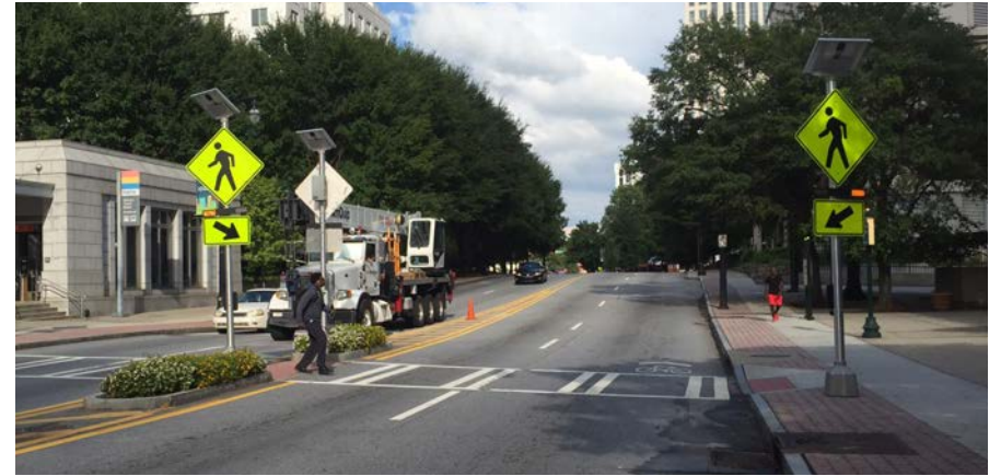
On multilane streets, multiple beacon installations are critical for awareness by motorists in all approach lanes.
