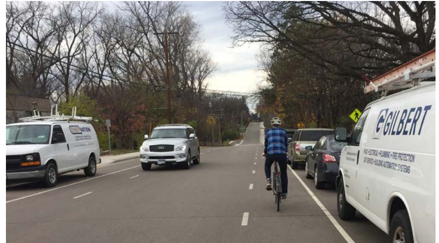
Advisory shoulders are located within the travel area, outside of any on-street parking lanes. Additional width should be allocated to the advisory shoulder area when configured adjacent to parking.
