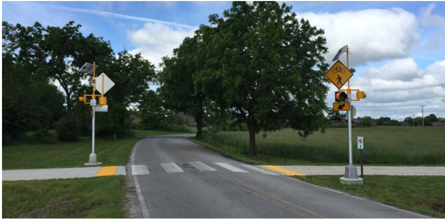
This path crossing includes many enhancements to slow traffic and promote yielding.
