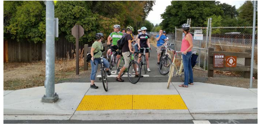
Along pathways with high volumes of users and at path crossings in highly developed areas with crosswalks, path crossings should provide adequate room for path users to wait outside of the path of crossing sidewalks.
