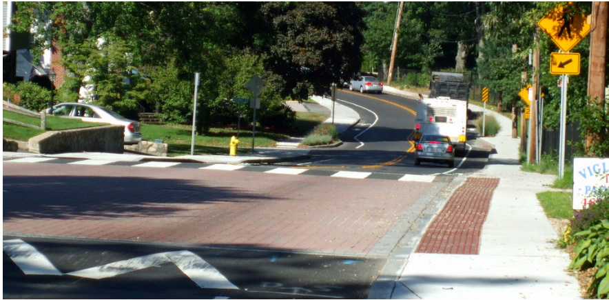
This trail crossing combines a median safety island with raised crosswalk.
