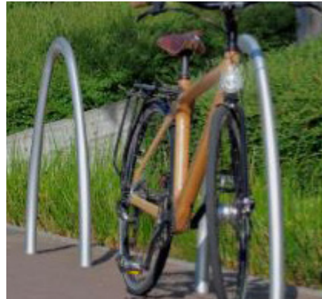
Minimum 4' spacing between racks
