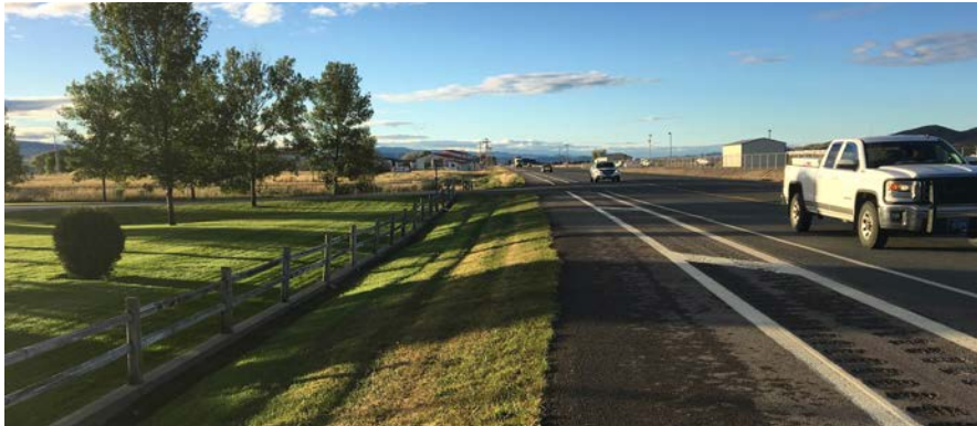
A wide paved surface, paired with a buffer area provides a more comfortable experience for bicyclists travelling on this shoulder.
