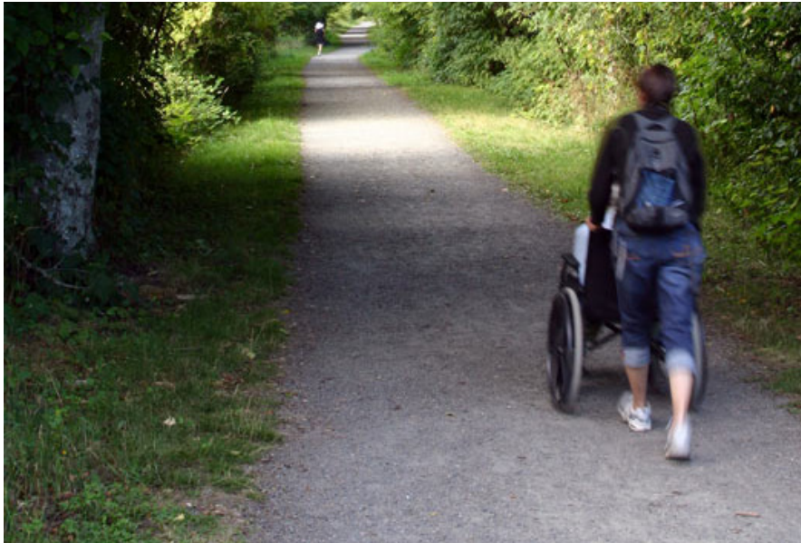
Smooth crusher fines can be a good surface material for natural surface trails for all user types (Source: National Trails Training Partnership)
