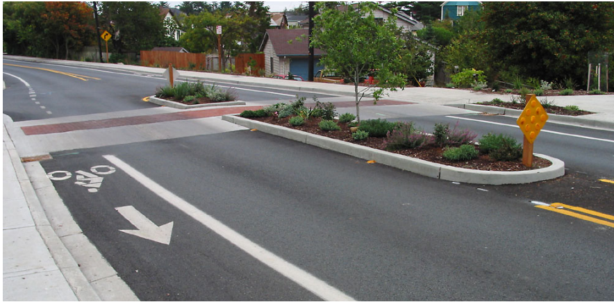
This midblock median refuge island and raised crosswalk allows pedestrians to cross the street in two stages.
