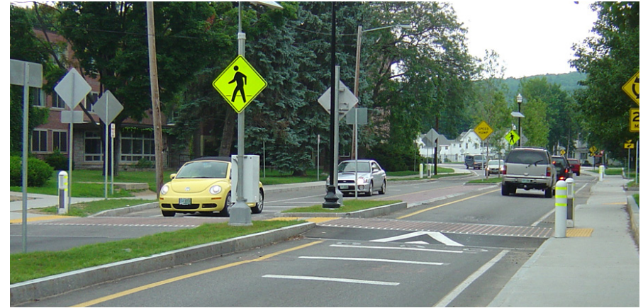
Raised crossings help to prioritize pedestrian movements across roadways.
