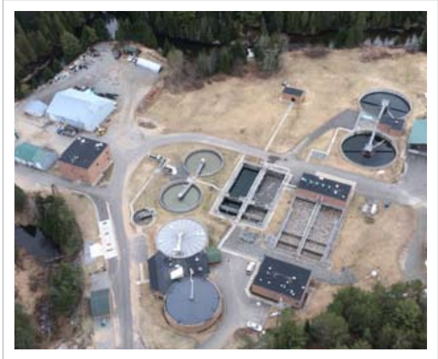
Aerial view of the Village of Lake Placid Wastewater Treatment Plant. Photo: Adirondack Council Staff
