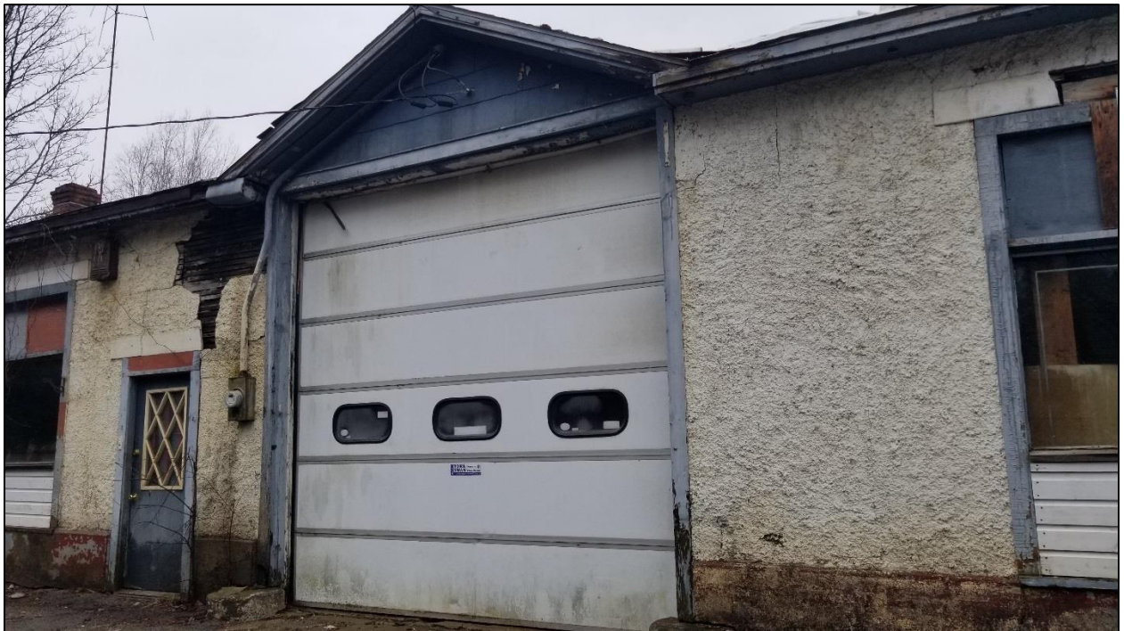
Photo 2. Building exterior facing Riverside Drive.
