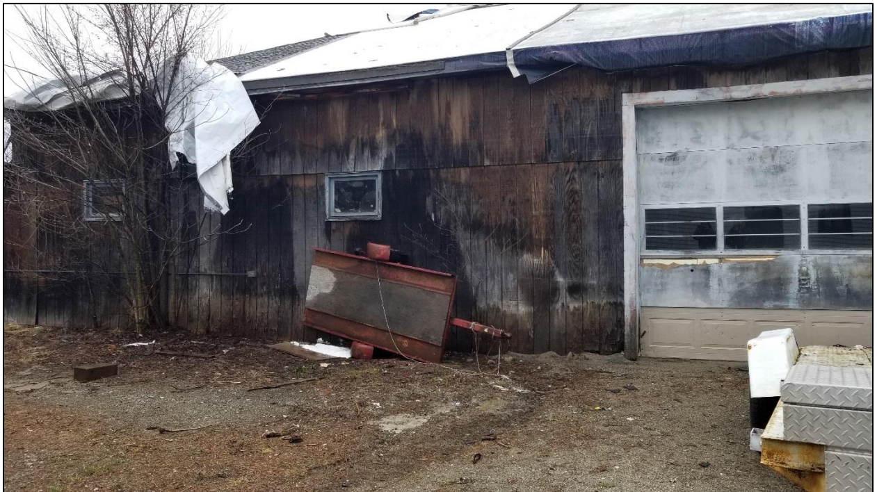
Photo 6. Eastern side of structure.
