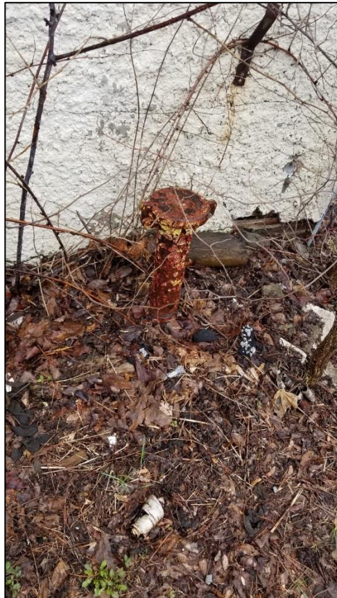
Photo 12. Yellow stickup pipe at eastern side of building – potential fill port.
