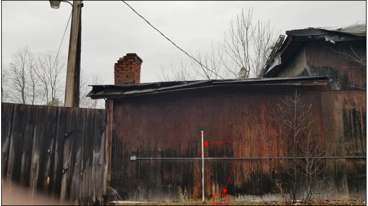
Photo 7. Eastern side of structure. Note potential fill port and vent.
