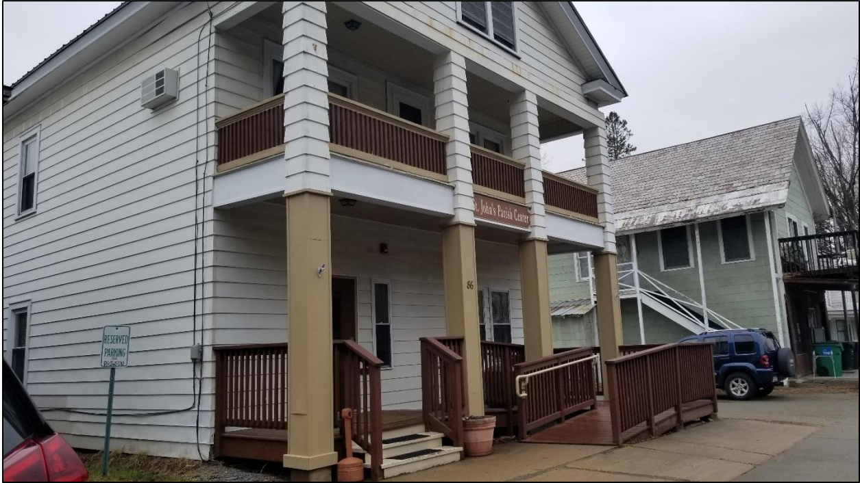
Photo 4. Looking west from building.
