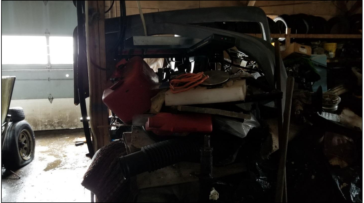
Photo 21. Piles of debris in main garage area.
