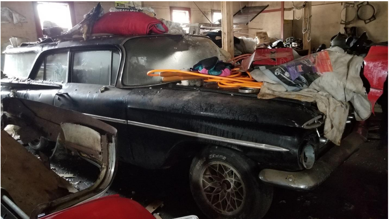
Photo 24. Old automobile and debris in main garage area.
