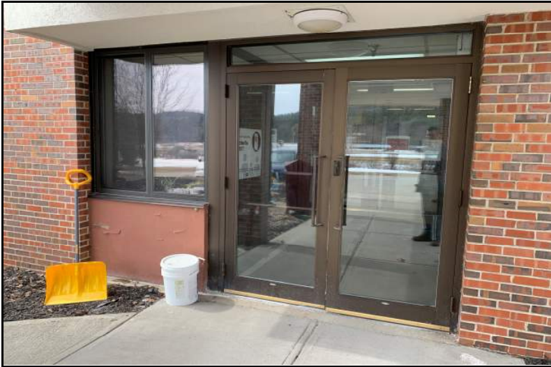
Photograph No. 7: Main entrance doors.
