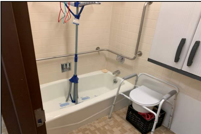
Photograph No. 25: Existing tub not currently utilized in Shower Room.
