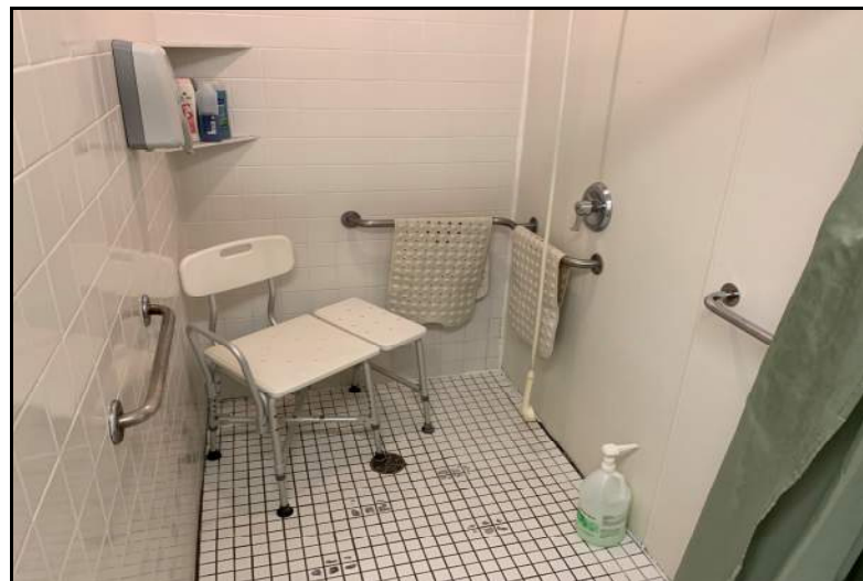
Photograph No. 24: Common Shower Room.
