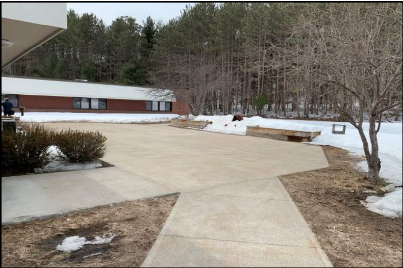
Photograph No. 9: Concrete patio west of dining area.
