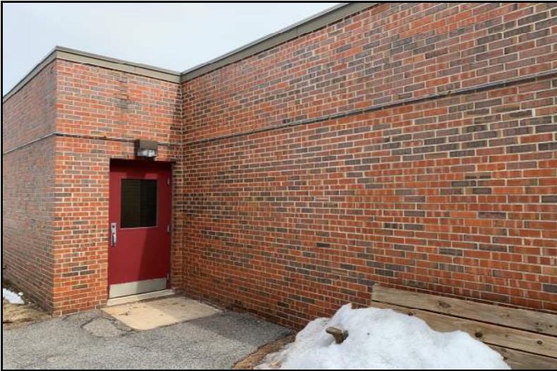
Photograph No. 8: Typical exterior door.
