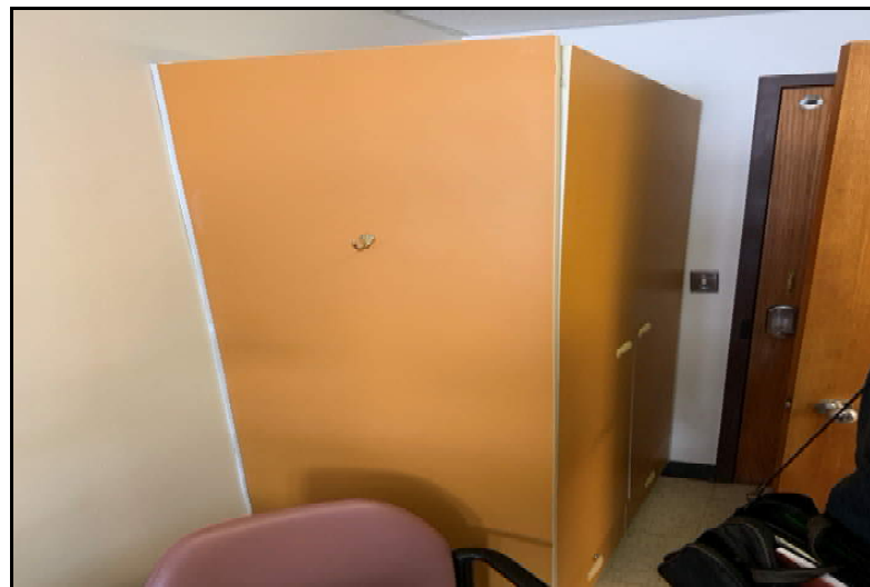
Photograph No. 20: Resident Room wardrobes
