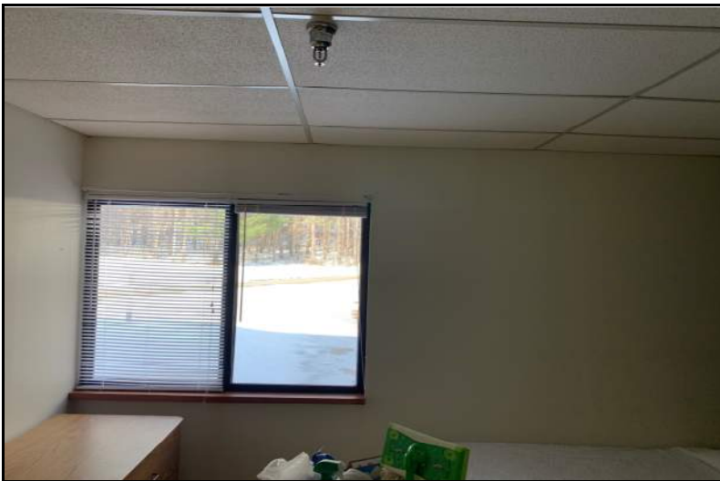
Photograph No. 17: Typical Resident Room.
