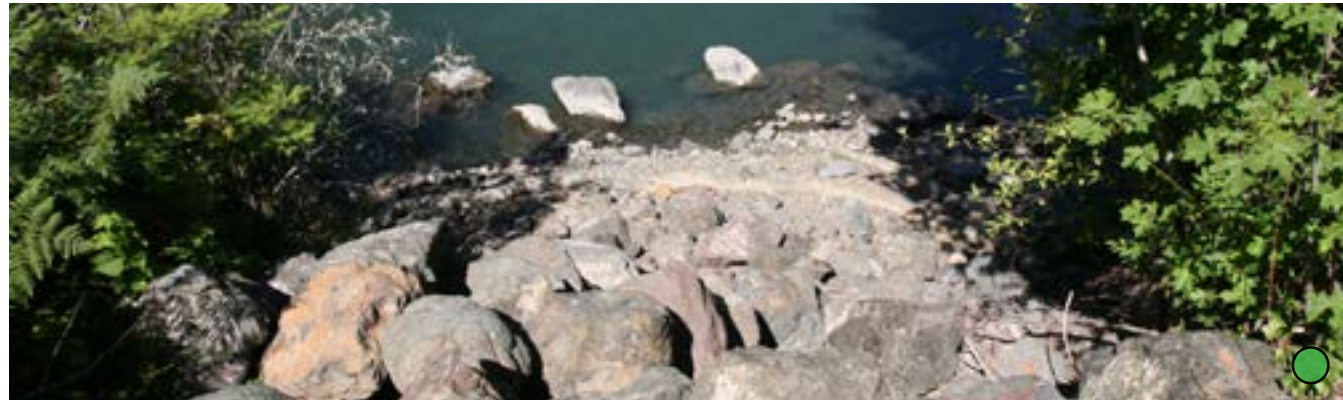
Riprap stabilizes the riverbank next to the existing bridge. This location provides uneven access to the river. The size of the riprap material creates a barrier to access for all but the most agile individuals. Credit: Thomas O'Keefe
