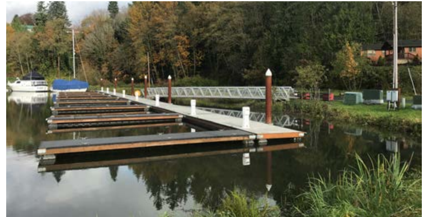
Existing gangway access to boat slips at along the north edge of the marina. Access to the gangway is from a paved road surface anchored by utility boxes, power poles and other infrastructure support marina activity. Credit: Jordan Sector
