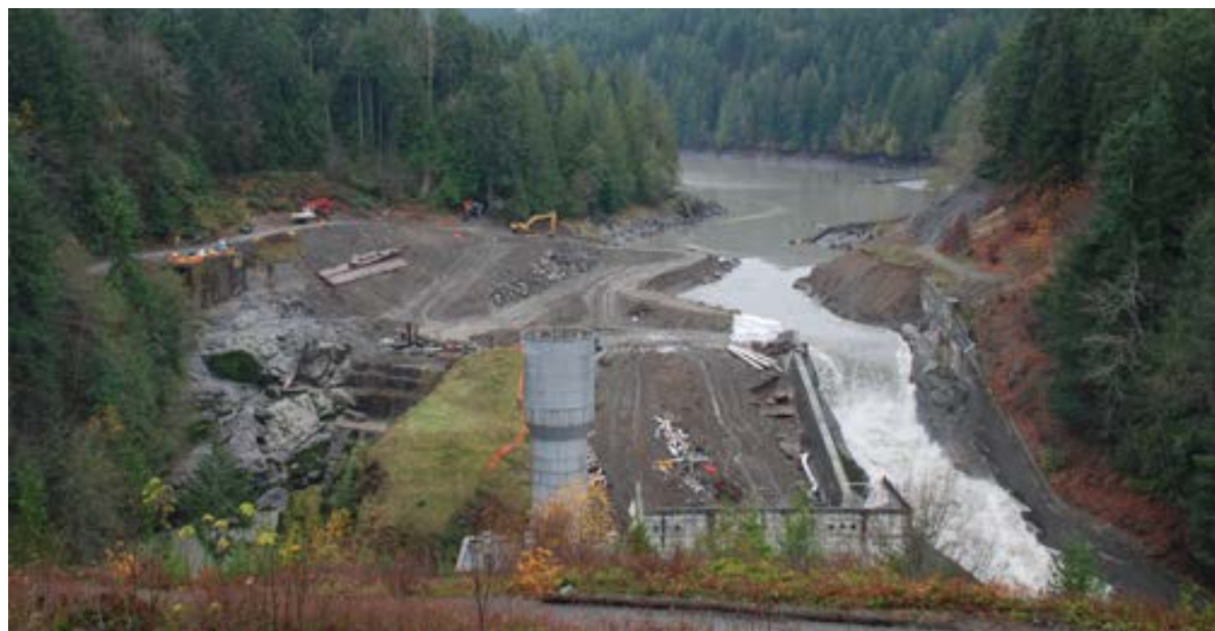
After a century of use for hydropower production, Elwha Dam removal began in the fall of 2011 and was completed within six months. With removal of the dam the reservoir transitioned to a river environment dramatically changing public access for rafts and kayaks who historically used access points on the upper end of the reservoir as take-outs for river trips. Credit: Thomas O’Keefe.
