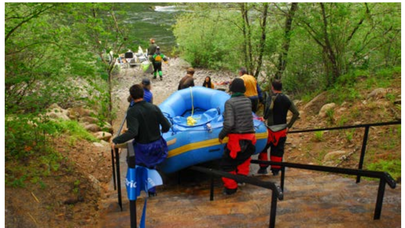
Rafters launching at Hole In The Wall, formally known as milepost 41. Site features include a boat slide and handrail system with a stamped-concrete staircase. The stair is designed to withstand high water flood events. Credit: Thomas O'Keefe.
