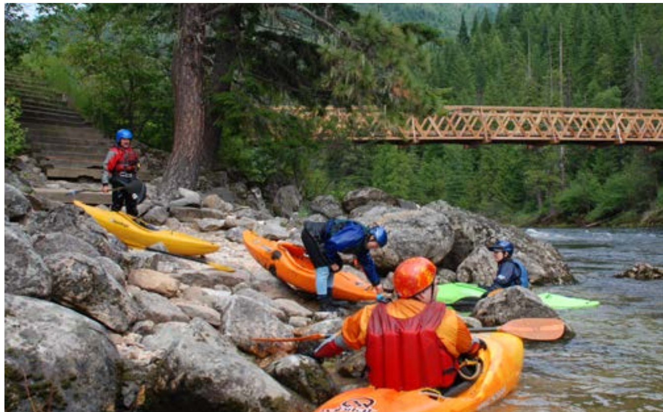
The Lochsa Wild and Scenic River in Idaho is a freely flowing, unregulated river. As a result, access is designed for a dynamic system where river levels can fluctuate widely. Steps at the Split Creek access end at the active channel, and boaters are required to navigate the last few yards through an area that is otherwise inundated at high flows. Credit: Thomas O'Keefe.
