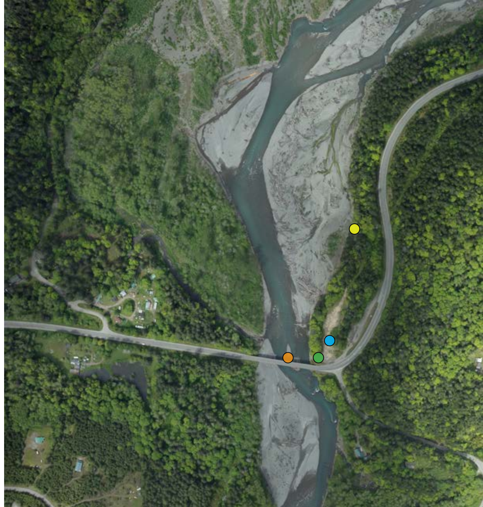
The Elwha River Bridge was built in 1926 and the 3-span, 388-foot, concrete-arch bridge has served the community over 90 years. Alluvial transport of sediments and significant change in river bed morphology have resulted in a river that flows below the bridge foundations.
