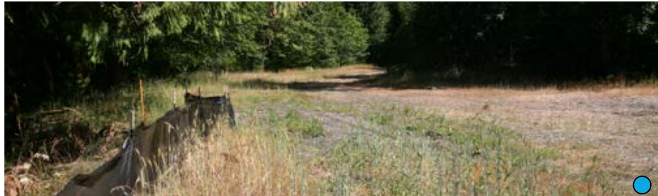
The existing site is clear of vegetation and used by Washington Department of Transportation as a staging area for materials. This site is at the centerline of the new highway and will link to the new bridge alignment. Credit: Thomas O'Keefe
