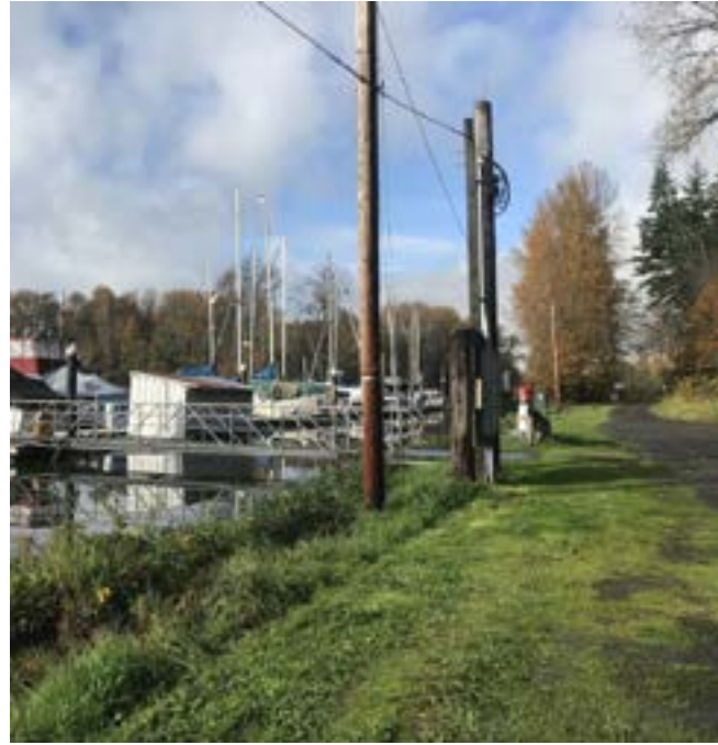
Parking area along the northern access road provides entry to the marina dock system. Marina utilities are secured at the top of bank and run along the the base of the gangway to the docks.
