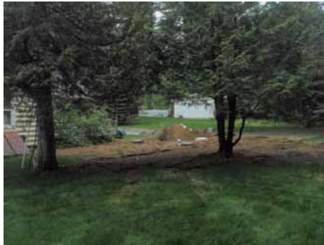
FIGURE 3-4 – Construction of an onsite wastewater treatment system in Lake George
