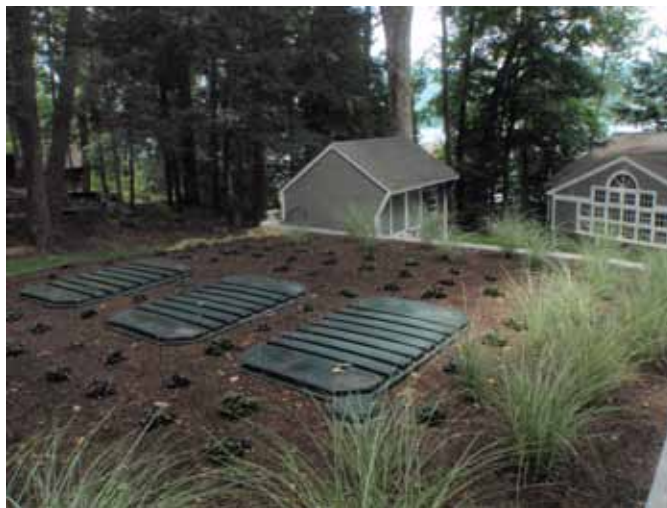
FIGURE 5-2 – Recent lakefront onsite wastewater treatment system
