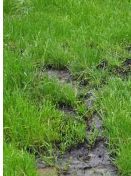
FIGURE 2-3 – Surfacing sewage indicating failing septic system
