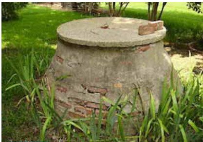
FIGURE 2-1 – Early Septic Tank
