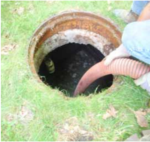
FIGURE 2-4 – Septic Tank Maintenance – Tank Pumpout
