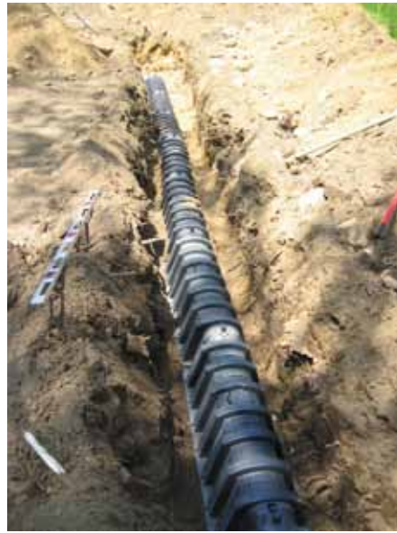
FIGURE 4-11 – Photo of installation of absorption field trench.
