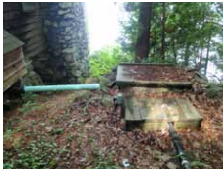
FIGURE 4-7 – Photo of an old system in the Town of Lake George
