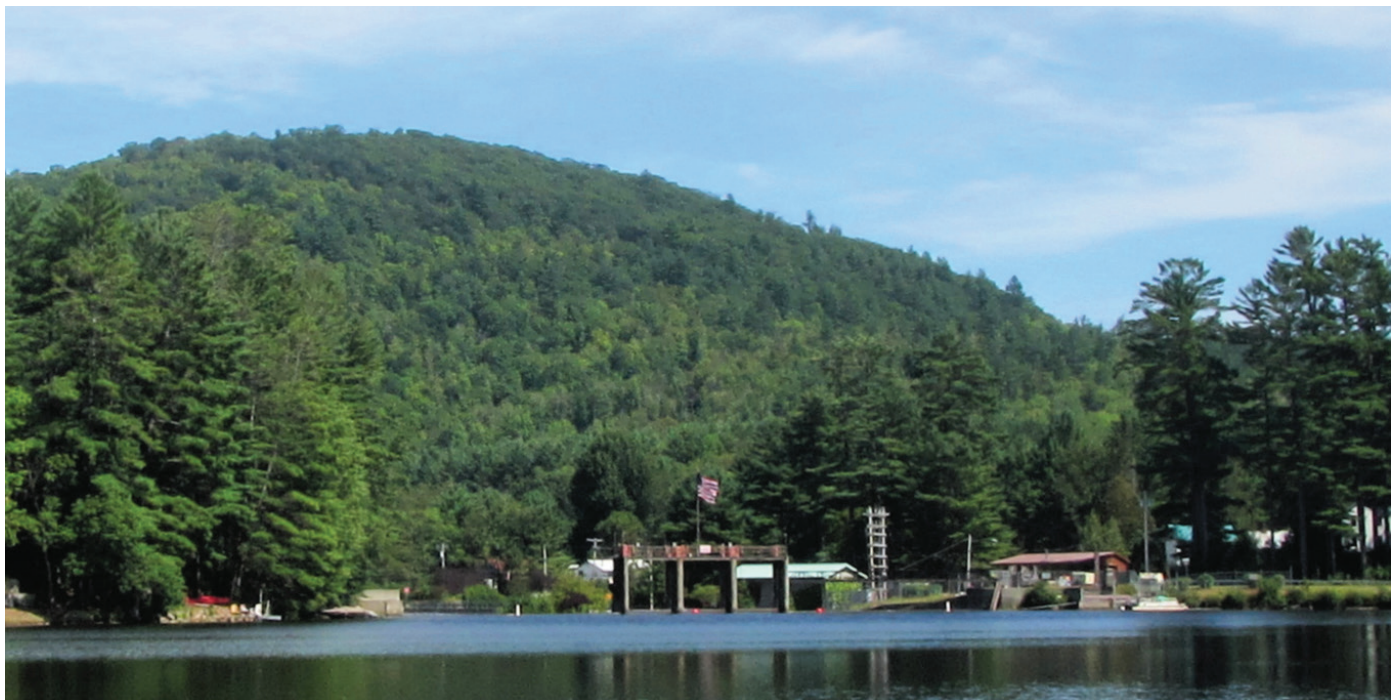
Photo 20: Lake Algonquin Dam is a Class C hazard rating dam in need of structural maintenance and repairs (Priority Project #P-06), Photo Courtesy of Caitlin Steward, Hamilton County SWCD
