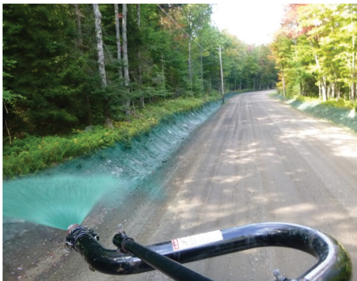
Photo 9: Hydroseeding prevents roadside erosion in Hamilton County.
