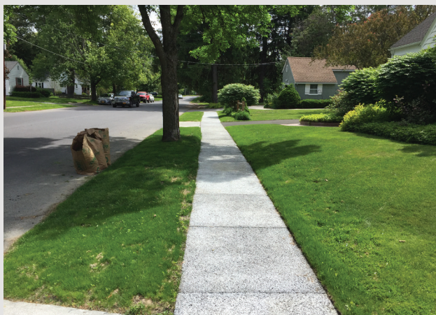
Photo 4: Completed porous sidewalk project, City of Glens Falls. Photo courtesy of Nick Rowell
