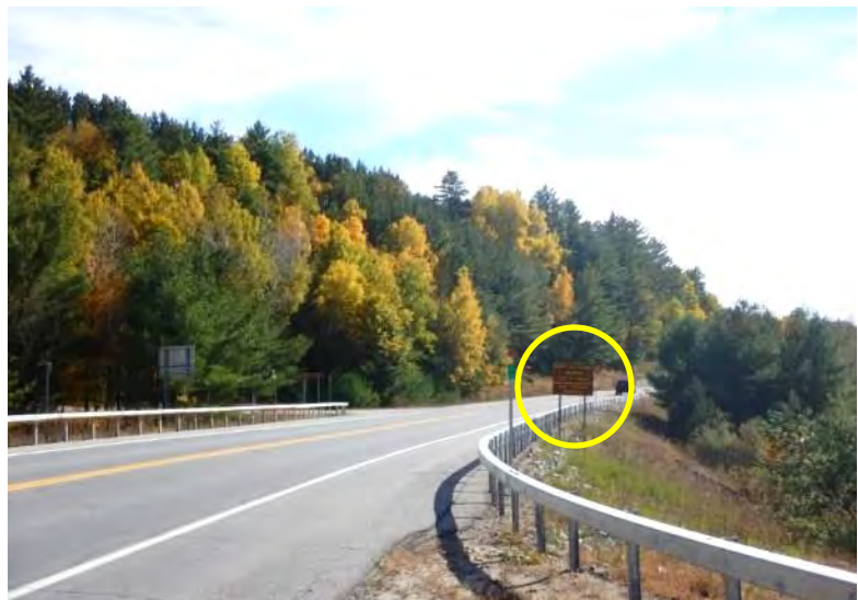
Figure 4 -- Intersection C Looking South, Sight Distance blocked by sign
