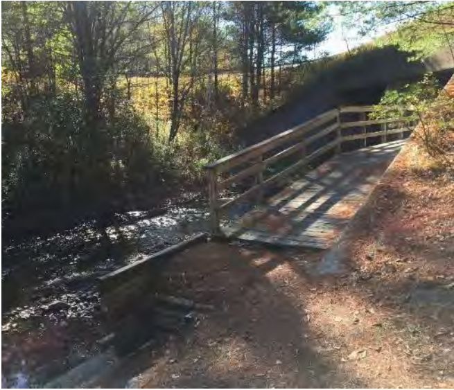
Figure 12 -- Pedestrian underpass, Carol Thomas Memorial Trail
