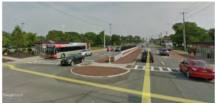
Figure 11 – Pedestrian Refuge Island
