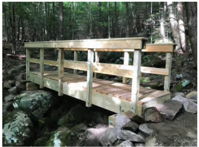
Above: 16-ft. pedestrian bridge with railing, Harris Land Preserve, Town of Luzerne, NY. Photo provided by Wilderness Property Management, Inc. [WPM].
