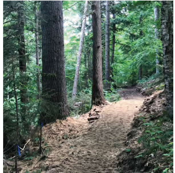
Above: Natural surface trail (bench cut with grade reversal alignment, College of Environmental Science and Forestry, Newcomb, NY. Photo provided by Wilderness Property Management, Inc. [WPM].
