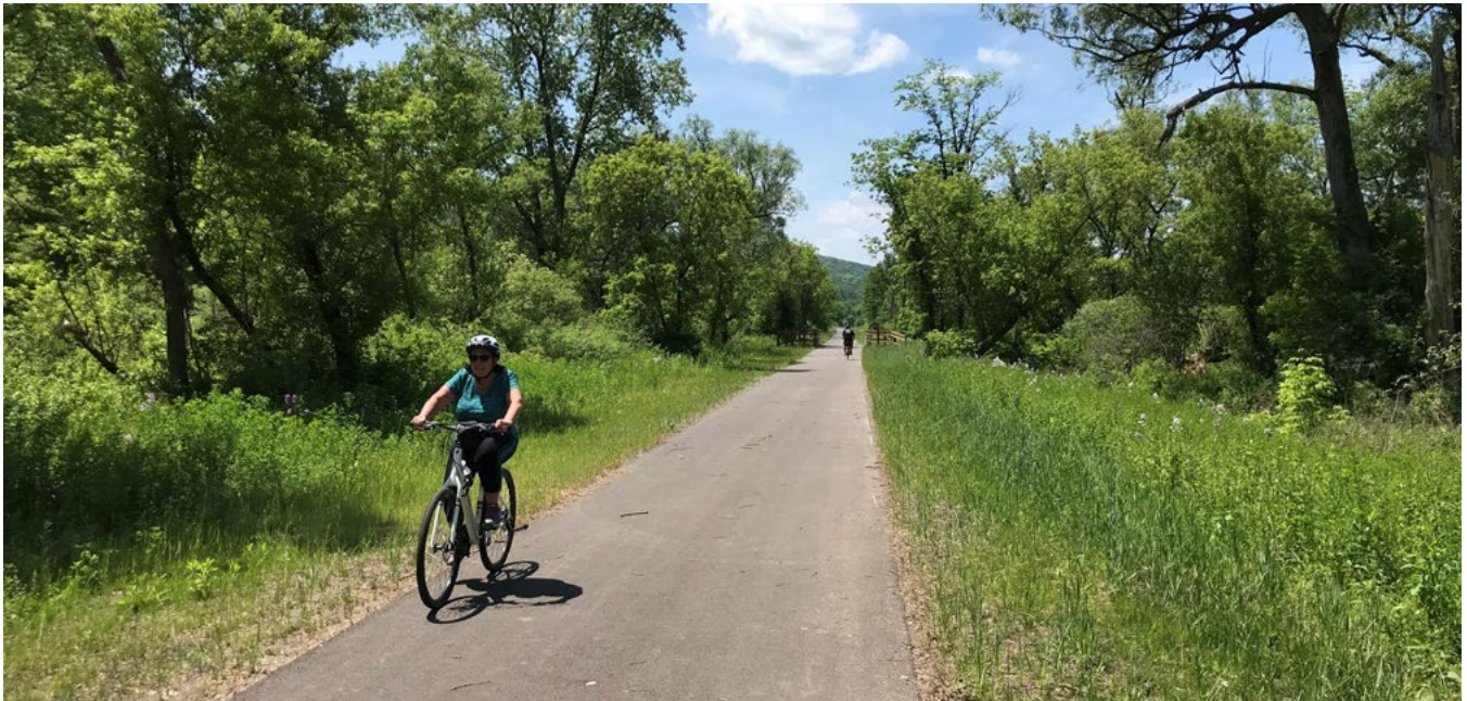
New trail constructed west of Little Falls in the Mohawk Valley.
