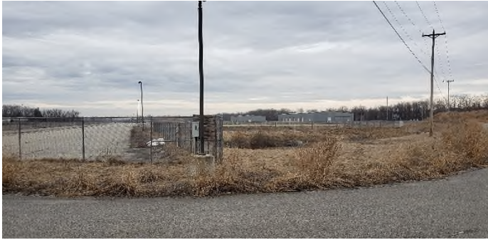
7.) Looking northeast, former dewatering areas and warehouses
