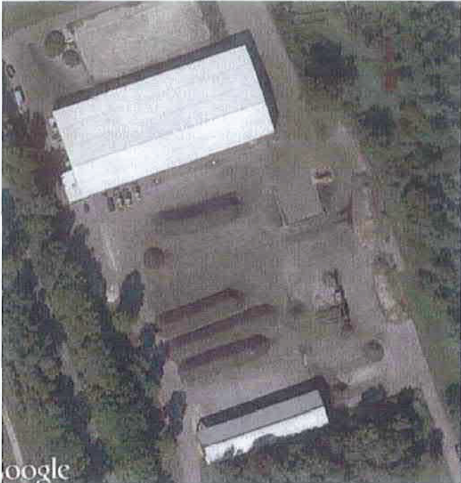
Outdoor windrow type Curing piles adjacent to enclosed Compost Facility (left). Typical Trommel Screen operation (below)
