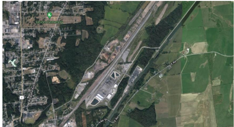
Figure 3-15 - Aerial View of Canalside Energy Park 2021
