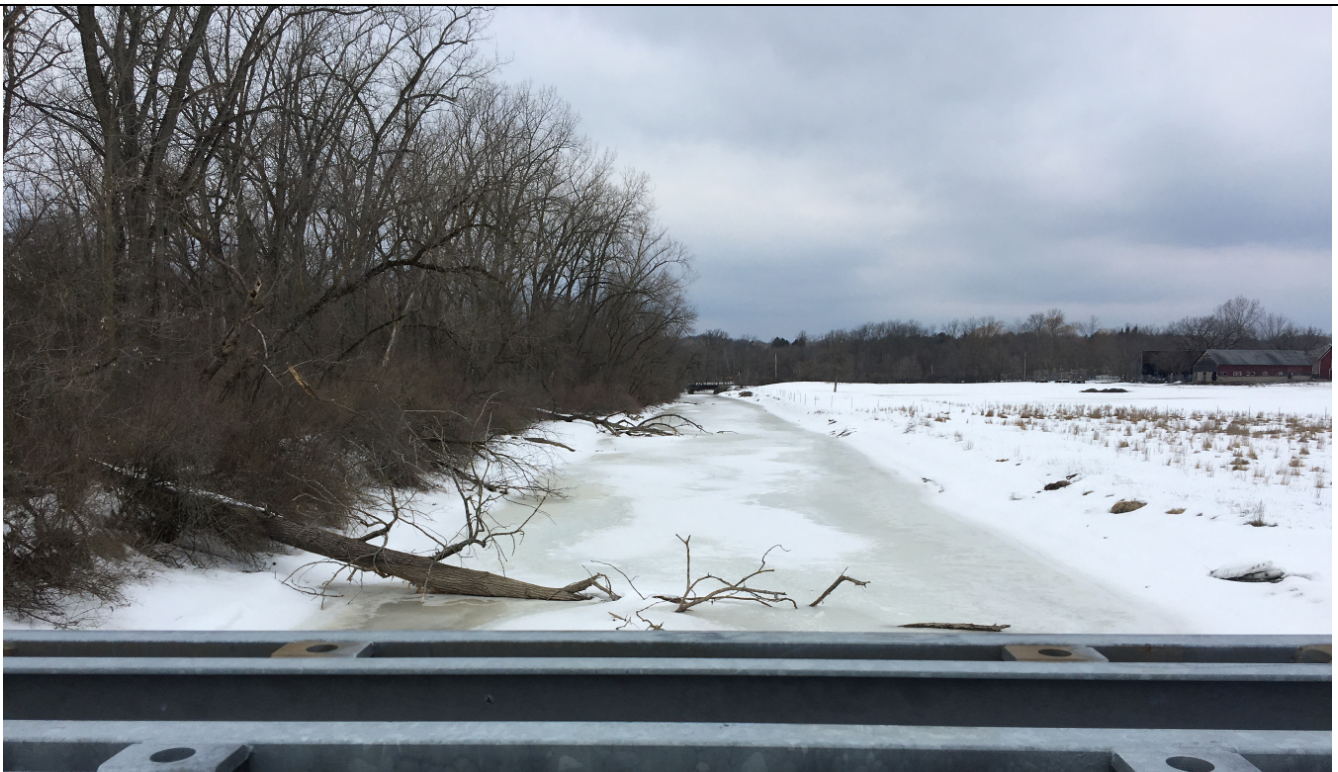
Photo 6 – Feeder Canal, looking west from bridge
