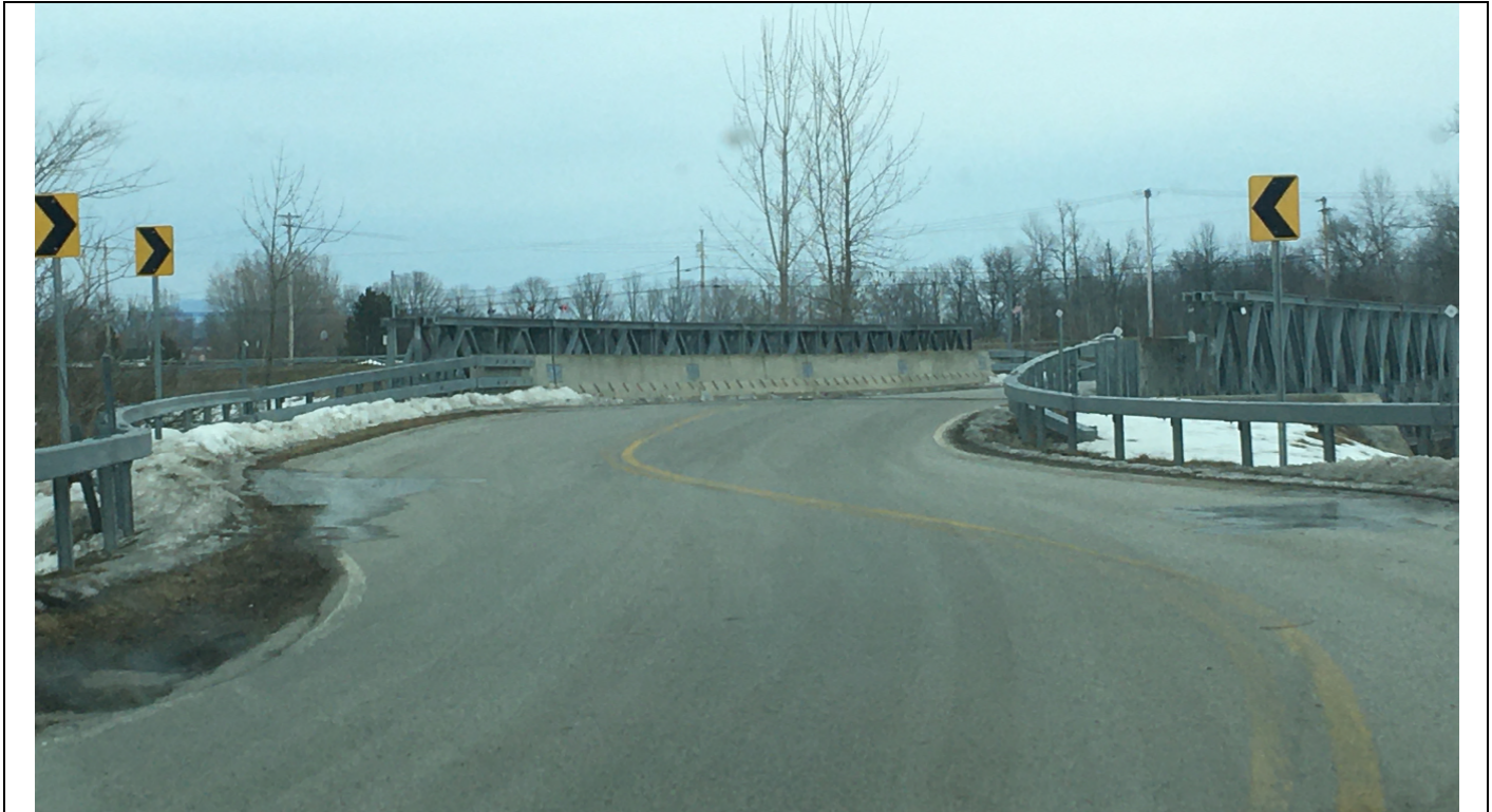
Photo 1 – South side Bridge Approach, looking north toward bridge
