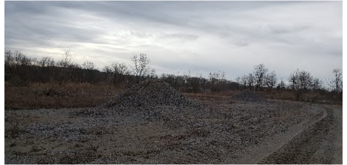
10.) Looking east, fill material pile
