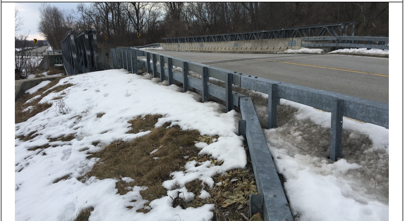
Photo 2 – North side Bridge Approach, looking south toward bridge
