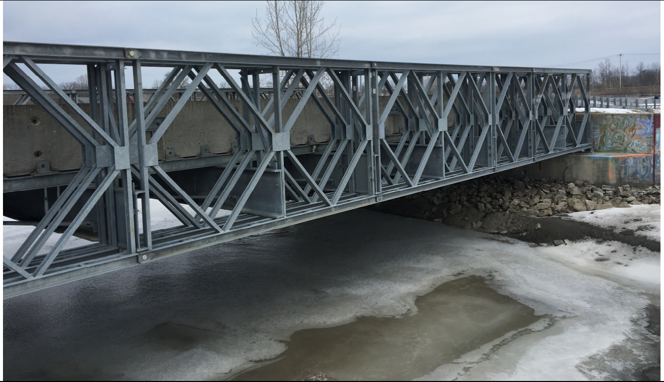
Photo 3 – East side Elevation of Bridge, looking west from southeast side
