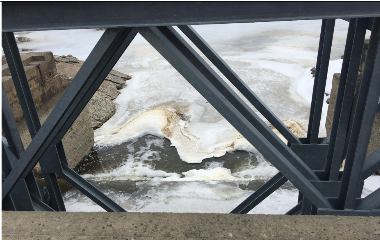
Photo 7 – Feeder Canal downstream from bridge, looking east
