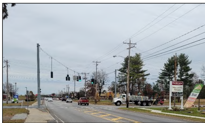
Photo #5 = Corinth Road/Big Bay Road Intersection
