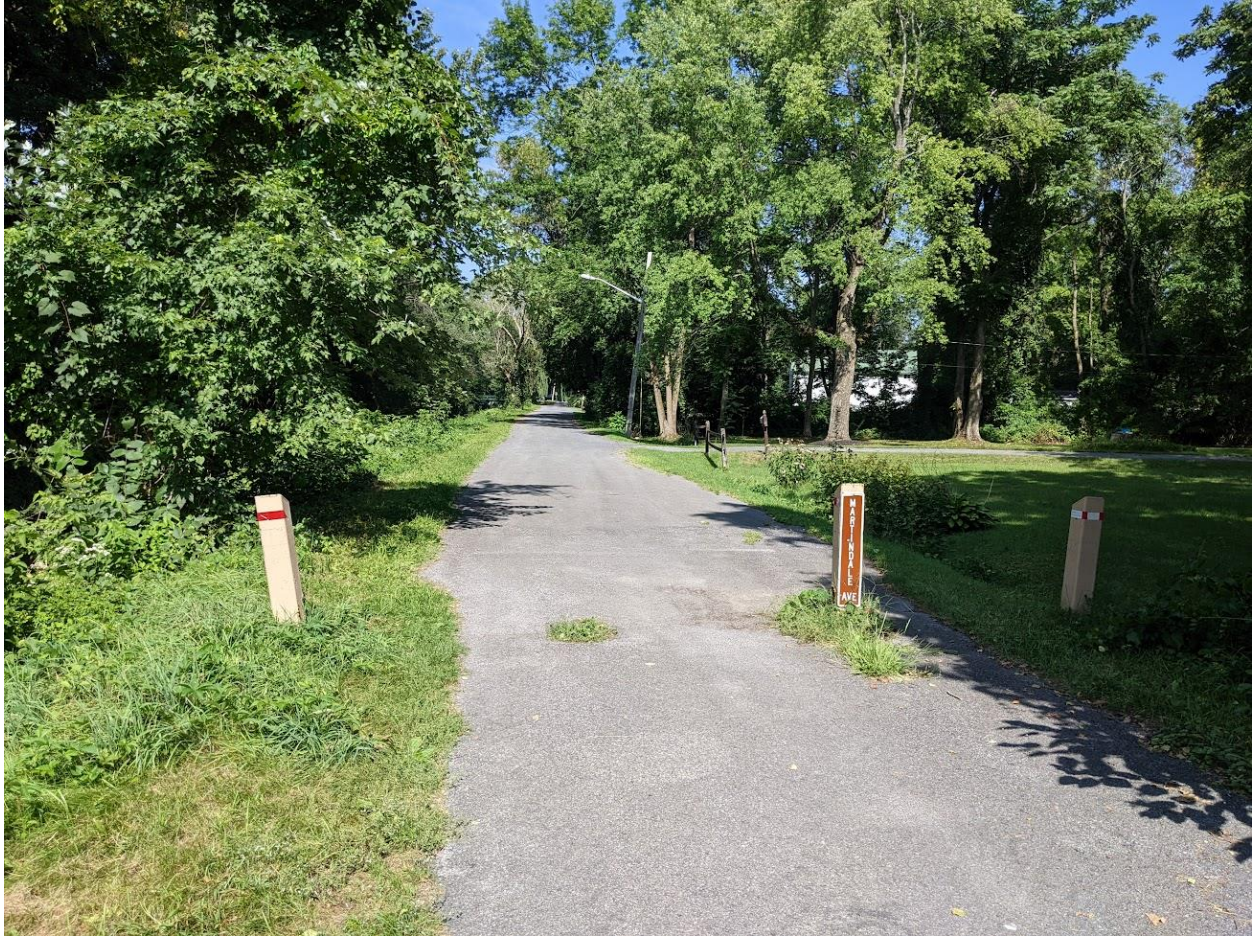
View looking westbound. When this picture was taken, the center bollard was removed leaving a large hole in the path to replace the bollard.
