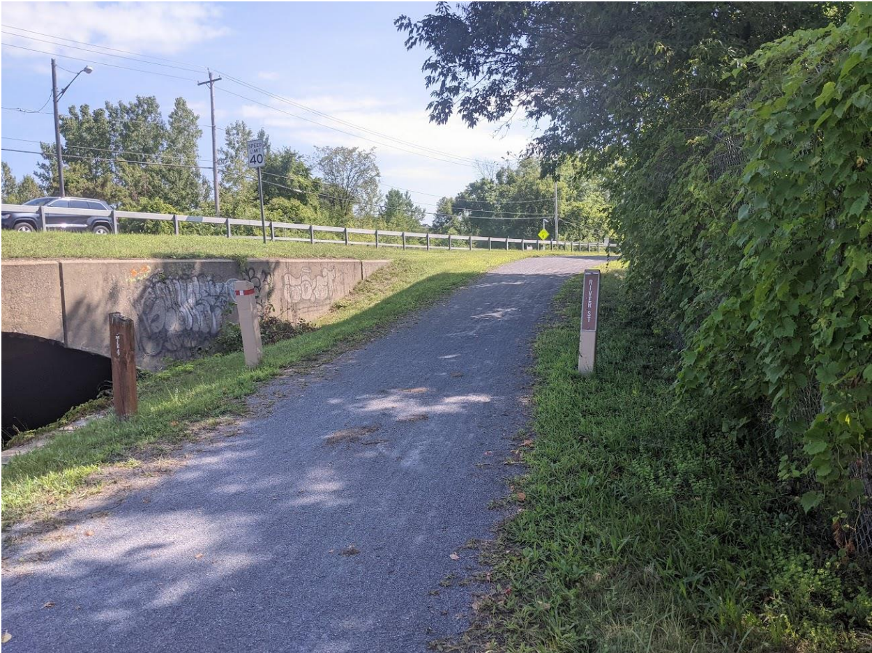
View looking eastbound
