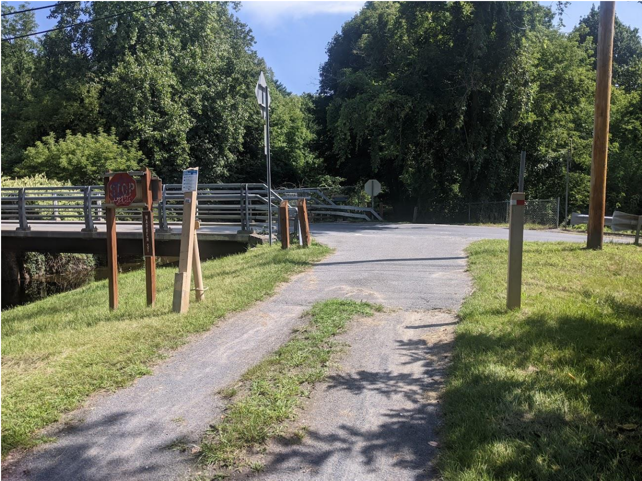
View looking eastbound
