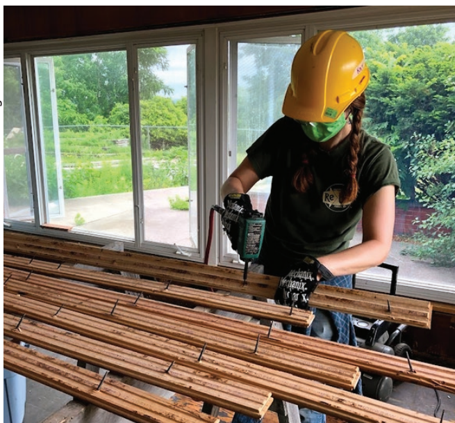
A volunteer removes nails from red oak flooring as part of a deconstruction project to recover reusable materials.
