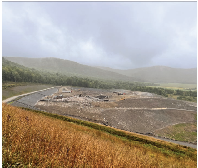
Municipal solid waste landfill in New York State
