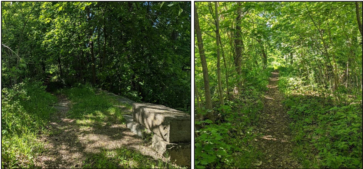
Figure 2-4: Existing Conditions of Adjacent Towpath
