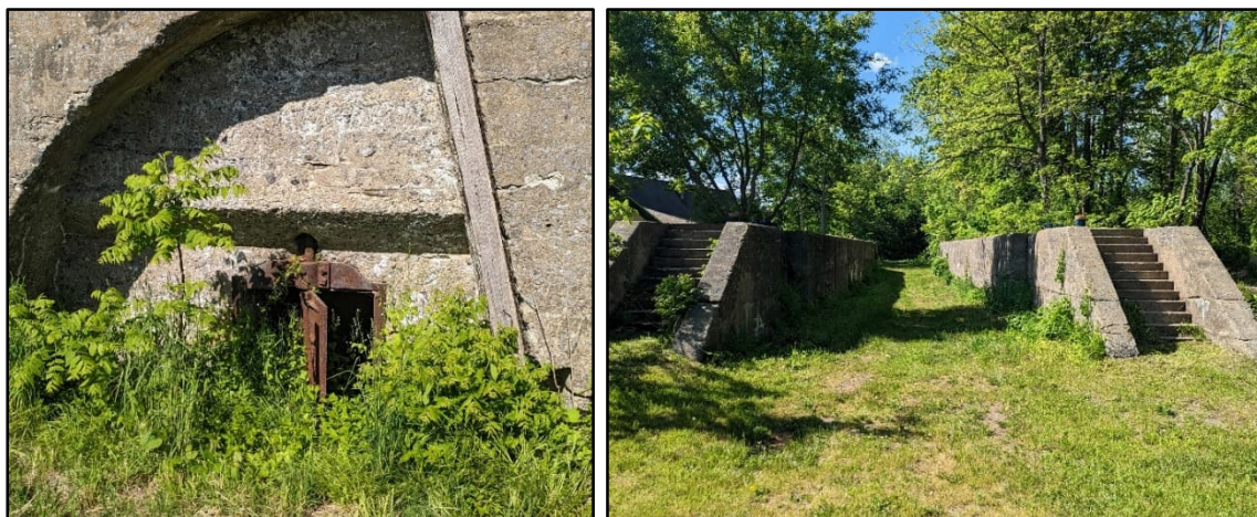
Figure 2-3: Existing Canal Junction Lock Infrastructure
