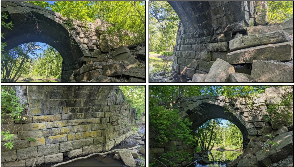
Figure 2-5: Existing Conditions of the Stone Arch Bridge
