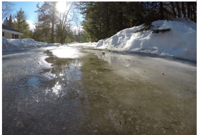
Figure 5.4.8-1. Warren County ice-covered Roadway, 2021
