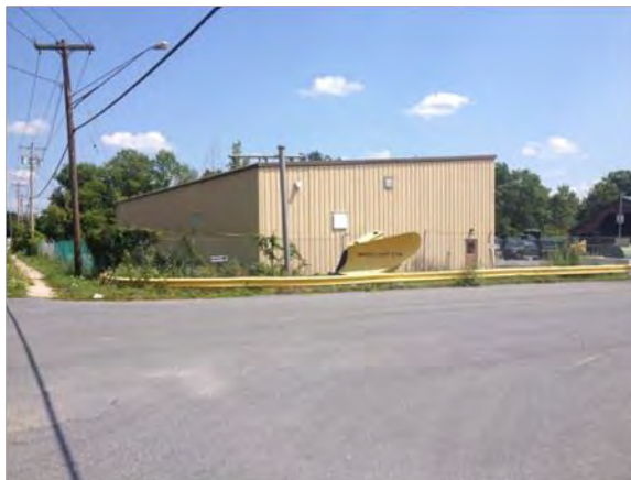
Warren County DPW Building on Lower Warren Street
