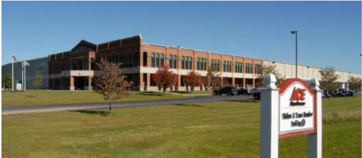
Entrance to Ace Hardware Distribution Warehouse on Ballard Road
