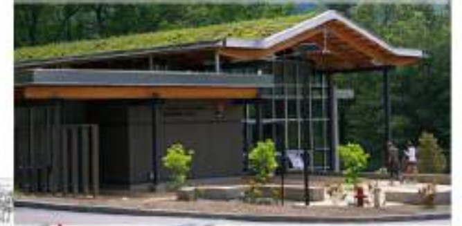
A visitors center with restroom facilities along the Feeder Canal Trail could help attract tourism.
