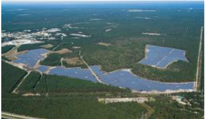
Aerial Image of Long Island Solar Farm
