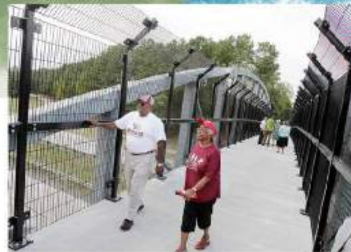
Pedestrian bridge over Canadian Pacific Railway can provide safe access to Hudson River waterfront and proposed recreational amenities.
