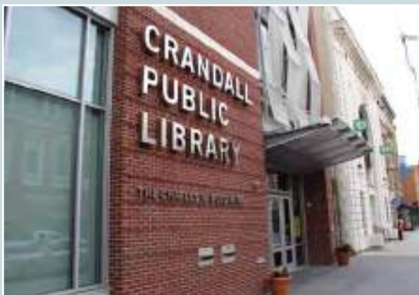
The renovated Crandall Public Library is LEED certified.
