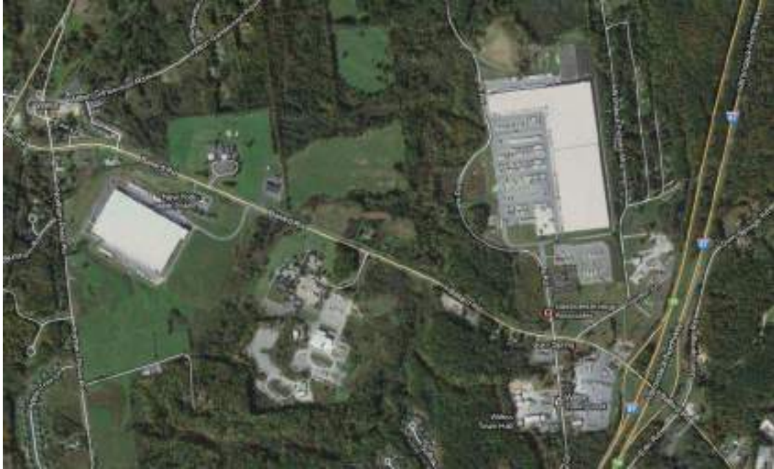
Aerial image of Ace Hardware Distribution located at the east, Target Distribution is located at the west. Wilton NY
