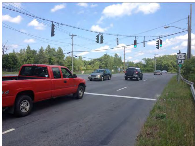
Lower Warren Street at Intersection with Quaker Road
