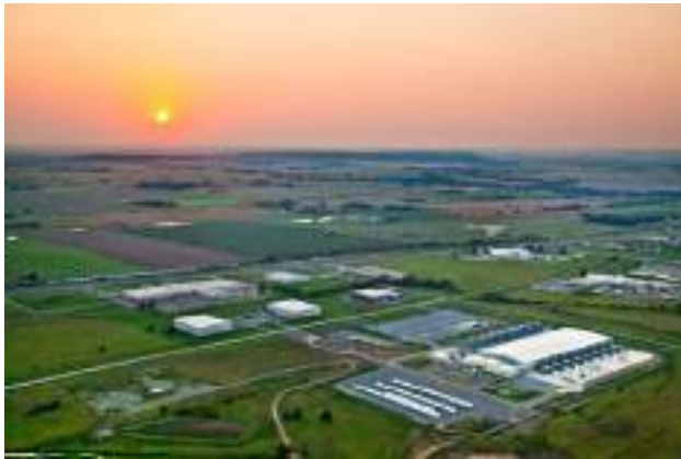
Aerial view of the Google Data Center in Pryor Oklahoma
