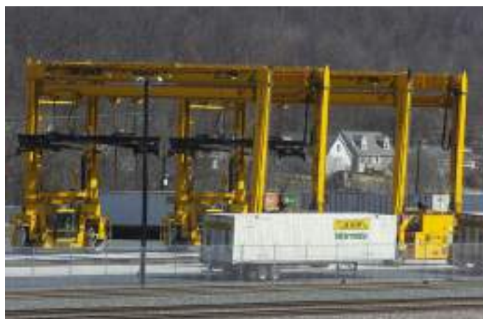
The transfer cranes at the intermodal facility
