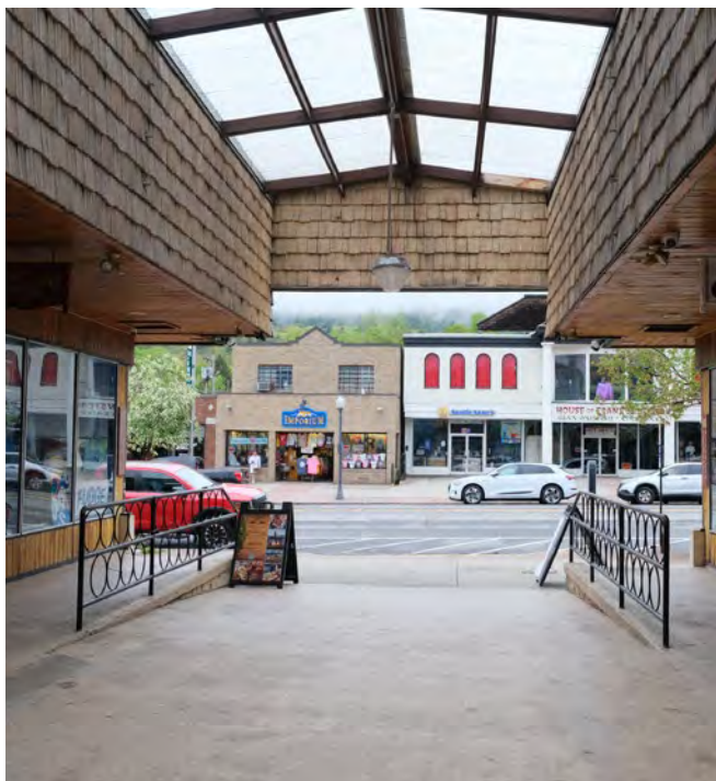
EXISTING VILLAGE MALL ATRIUM - CANADA ST
