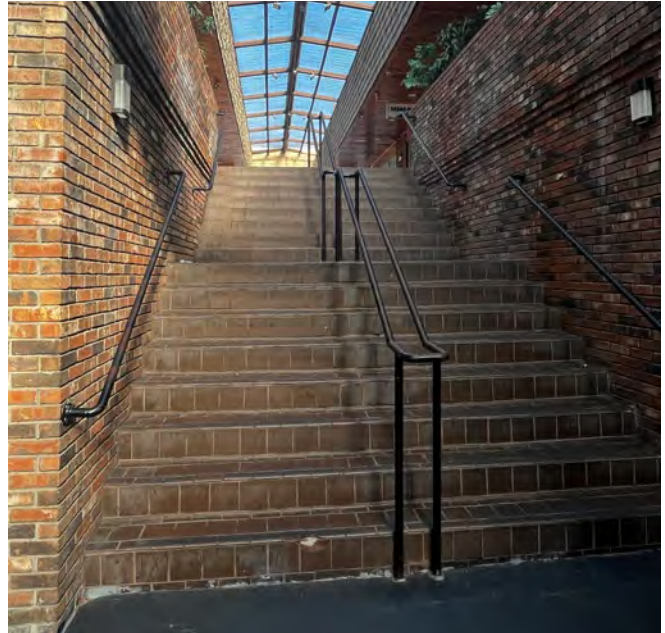
EXISTING MALL INTERIOR STAIRS
