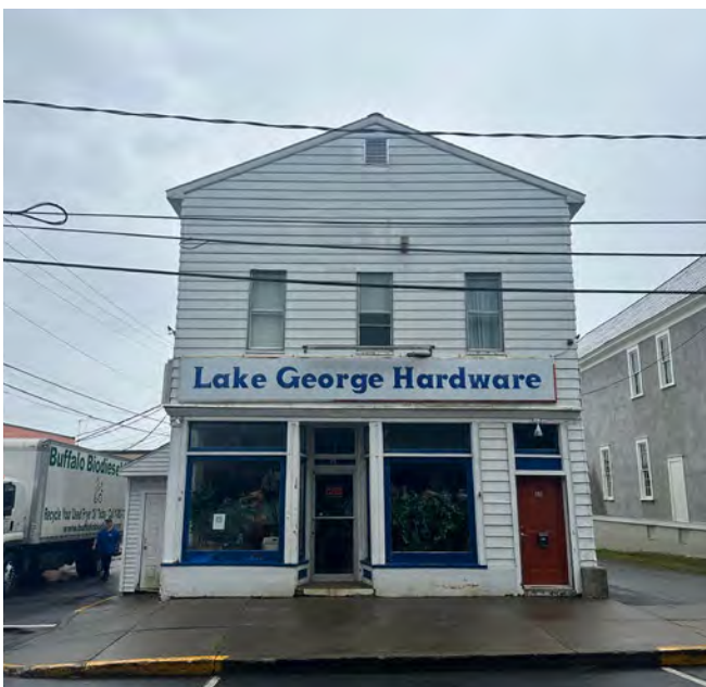
EXISTING EXTERIOR FRONT FAÇADE ALONG MONTCALM ST
