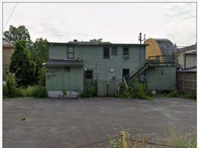
EXISTING REAR FAÇADE AND PARKING LOT CONDITIONS
