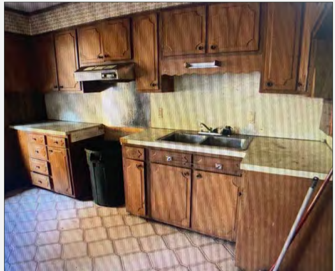
EXISTING SECOND FLOOR KITCHEN
