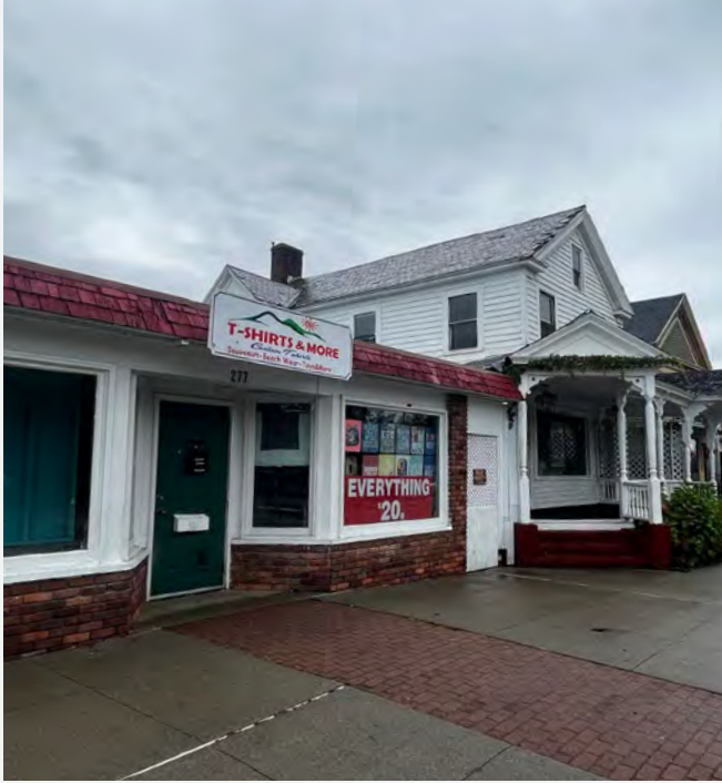
EXISTING STRUCTURES AT 277 AND 279 CANADA ST
