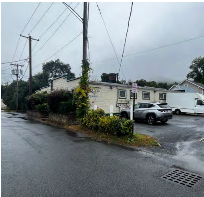
EXISTING WAREHOUSE APPROACH - IROQUOIS ST
