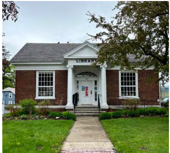
EXISTING LIBRARY ENTRANCE ALONG CANADA ST
