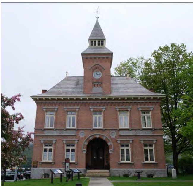
EXISTING BUILDING FAÇADE ALONG CANADA ST
