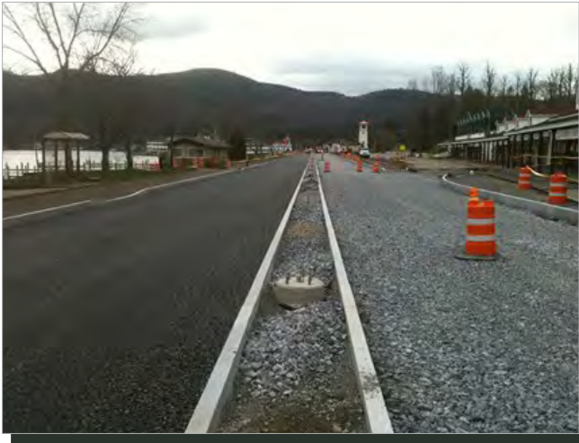
BEACH ROAD DURING POROUS PAVEMENT INSTALLATION (IMAGE CREDITS: PROTECT THE ADIRONDACKS, AUGUST 2013)
