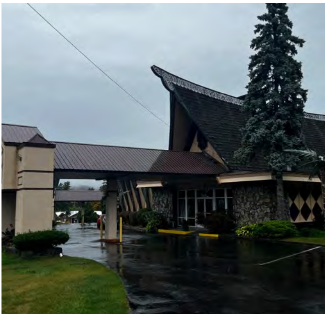
TIKI HOTEL - FACADE RENOVATION PROJECT
