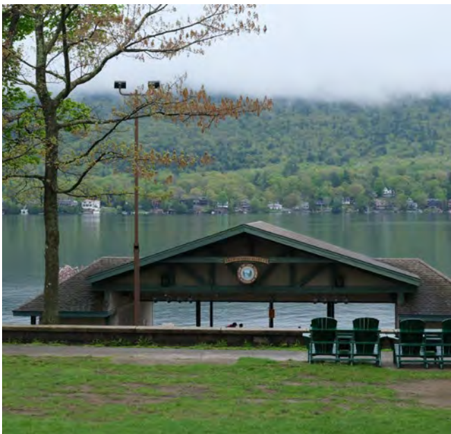
PREVIOUS SHELTER PRIOR TO FIRE OF SUMMER 2024
