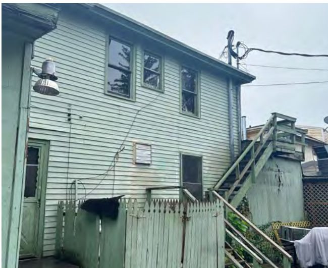
EXISTING EXTERIOR STAIRWAY TO SECOND FLOOR
