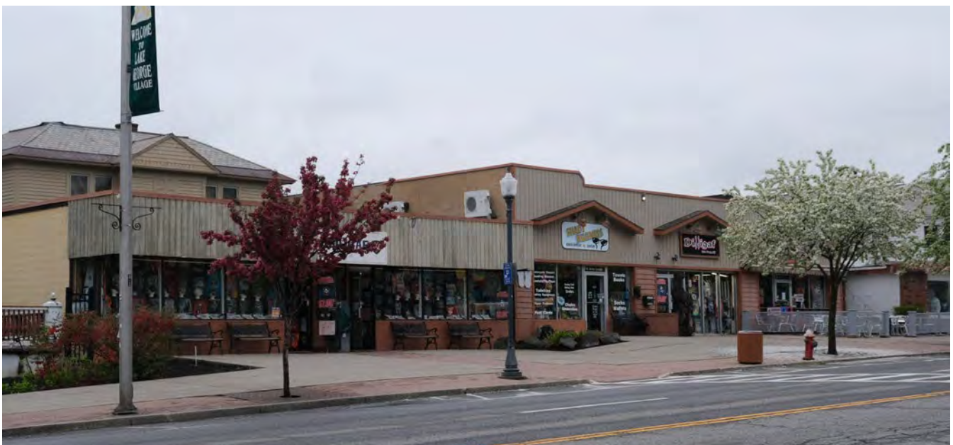
STOREFRONTS ALONG CANADA ST
