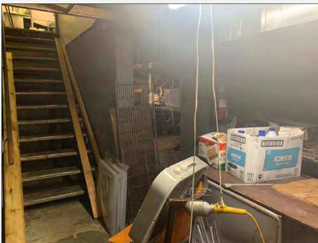
EXISTING BASEMENT LEVEL CONDITIONS
