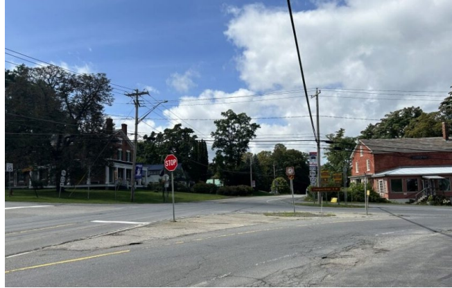
Photo 9: The focus area's northern gateway is defined by a confusing intersection and unclear signage. Photo Source: LCLGRP.
