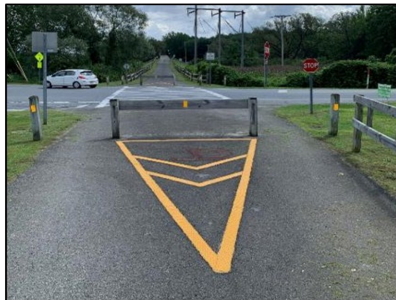
Figures 4-1 and 4-2: Above: The Barrier, or Fence, Installed at Several Locations along the Bikeway. Note the Inadequate Lane Width.
