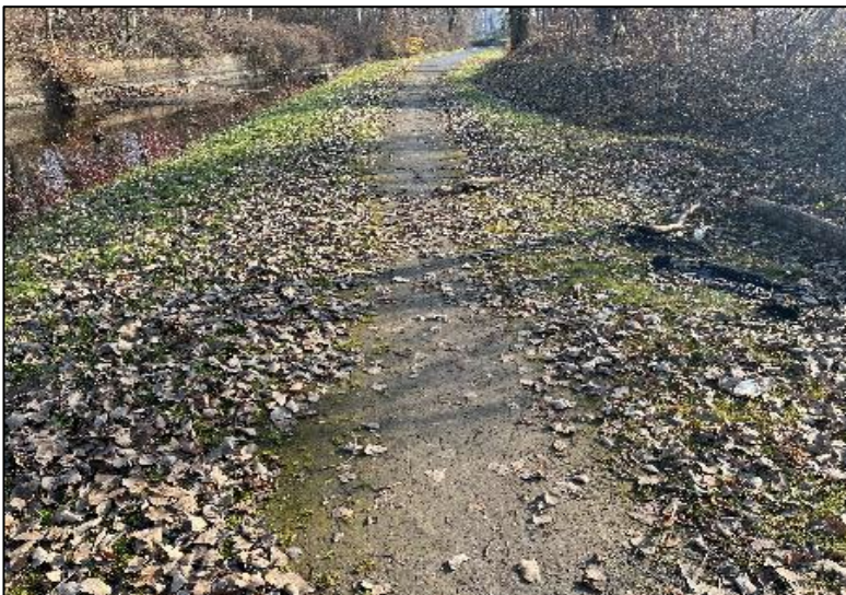
Figure 3-33: Example of Trail Surface Washout.
