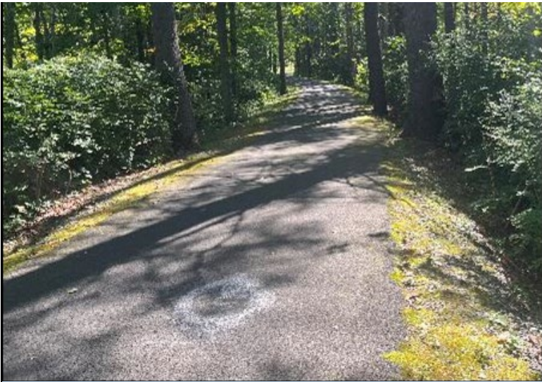
Figure 3-17: Pothole and Moss Growth on the Bikeway.
