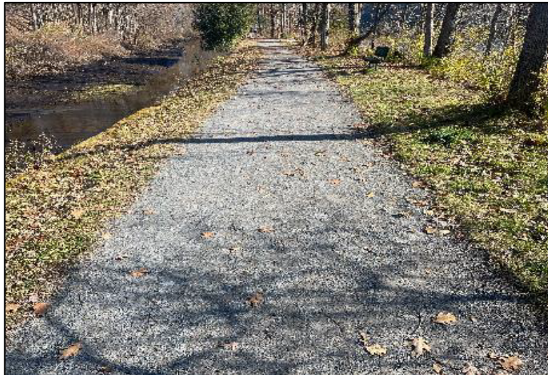
Figure 3-26: Typical Stone Dust Trail Adjacent to Feeder Canal.
