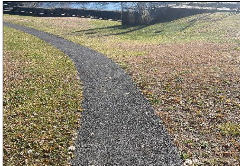
Figure 3-25: Four-Foot Wide Asphalt Path Through Overlook Park.
