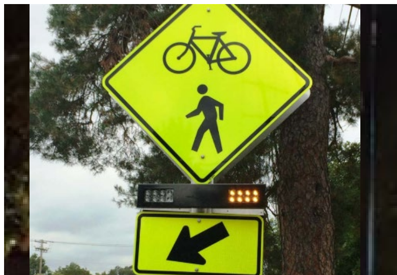
Figure 4-5: Example of a RRFB. Source: Universalsigns.com.
