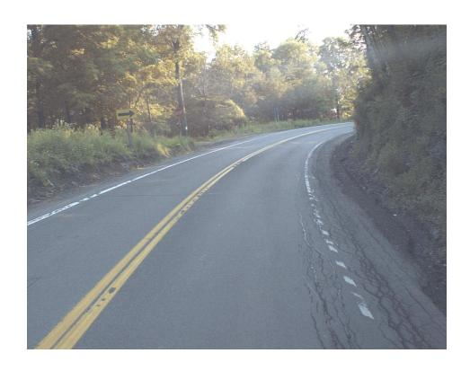
The distress is identified as "high" severity (photo at right) when the effect of the height difference can be detected when driving across the drop, or has the potential to influence the track of a vehicle.
