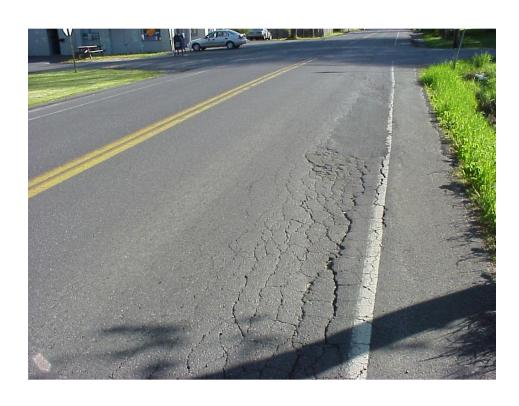
The longitudinal crack in this photo qualifies as alligator cracking even though it lacks the interconnected cracking. The crack is in the early stages of development, but still represents a load-related distress because it occurs in the wheelpath.
