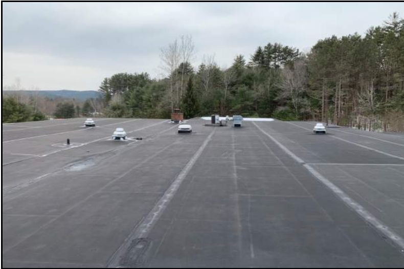
Photograph No. 11: Existing EPDM roofing.
