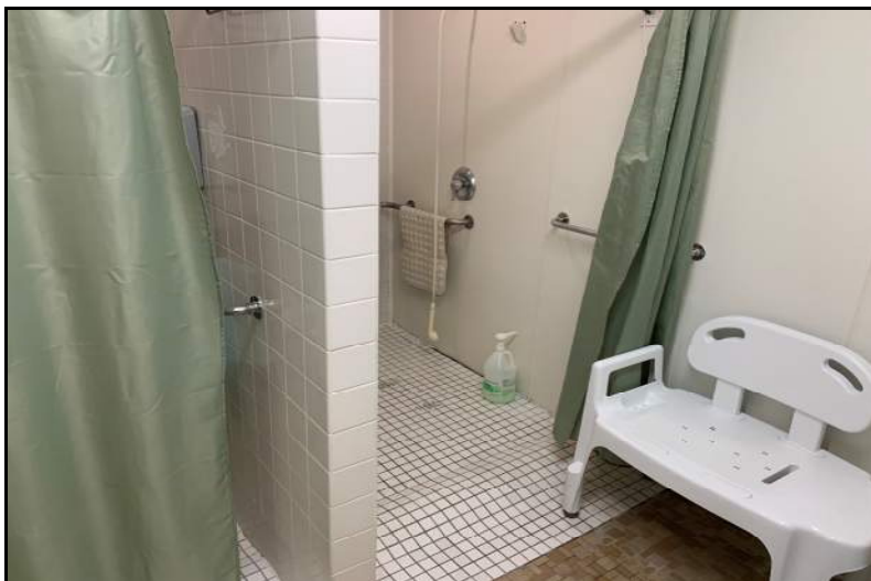
Photograph No. 23: Common Shower Room.
