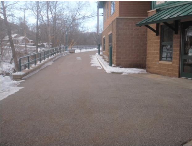
The rear of the building where ADA access is available.
