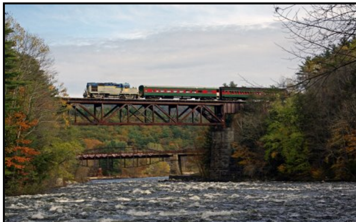
Figure 14: Hadley/Luzerne Trestle (foreground) 90 feet above the Sacandaga River at the confluence with the Hudson River. The landmarked Parabolic Bridge in background. Both illustrate the marvels of 19th Century engineering. Courtesy of G. Klinger.
