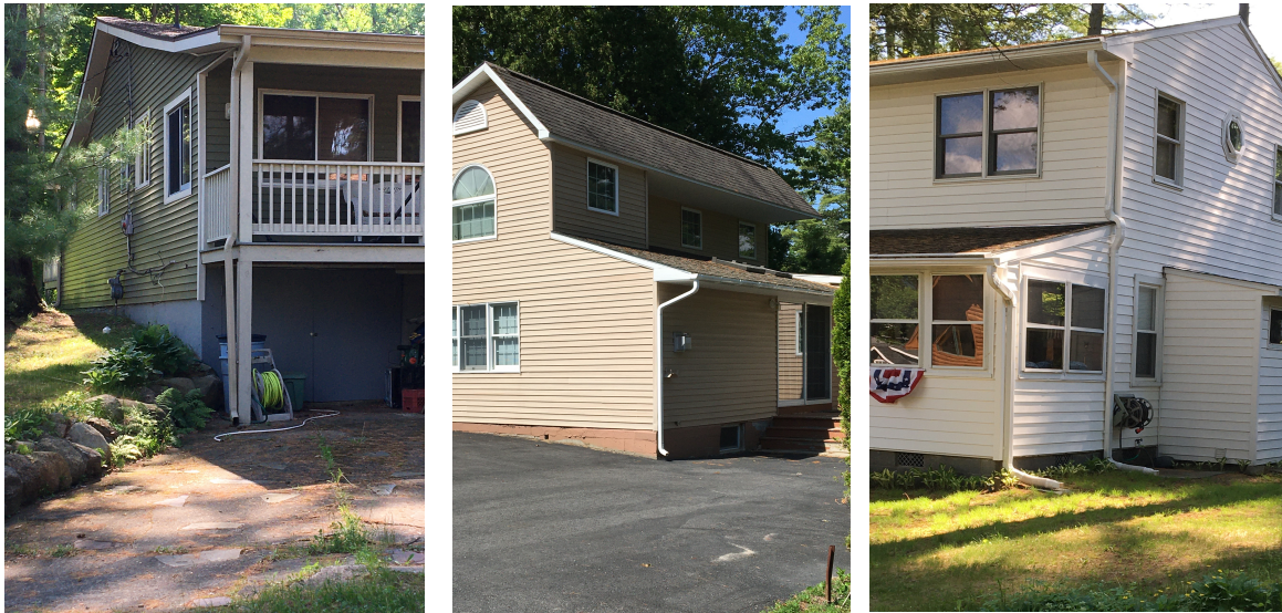
Figure 2. Downspouts that connect to impervious areas (left two photos) versus disconnected downspouts (right).
