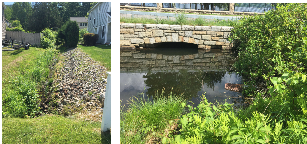
Figure 4. Western end of swale running between residences located off of Cedar Lane (left), culvert outlet in wetland, with Lake George in background (right).
